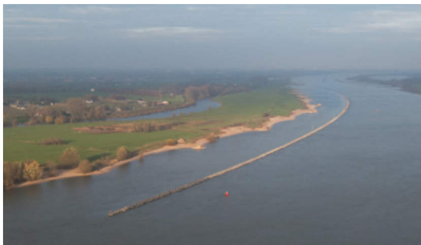
Figure H.2: Longitudinal dam in the river Waal (Buijse, 2015).
