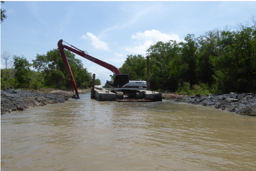
Figure K.6: Dredging practices in one of the channels in the Ciénaga Grande (September 20, 2017).
