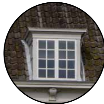
Dormers, combination of wood and plumbum
