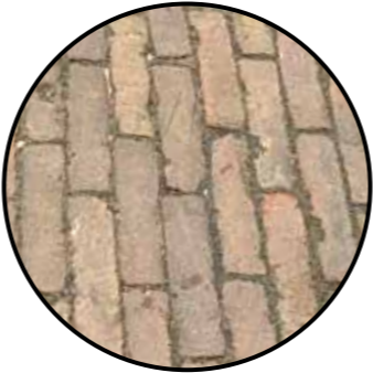
Pavement south square
