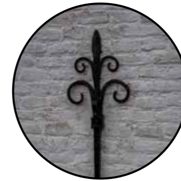
Wrought iron wall anchors
