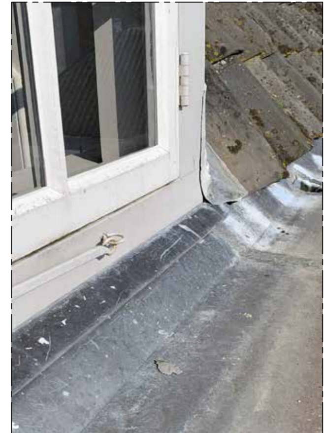
photo of dormer window and gutter
