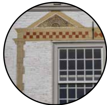
Wooden windowframes with sandstone ornamentation
