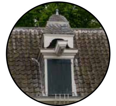
Wooden lifting hatch with slated roof
