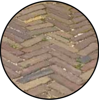
Pavement south square
