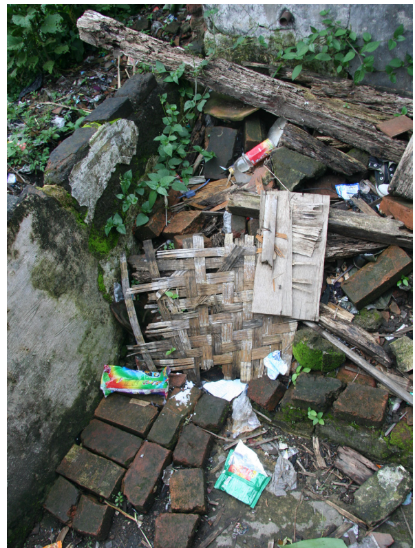
Figure 12: Debris and rubble sorted from the re-usable salvaged bricks. Source: own image
