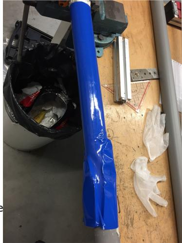
(b): The shrink sleeve is pulled over the impregnated glass fibre sleeve.
