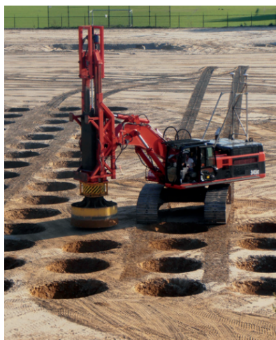
Figure 2.3: C.D.C. in progress
