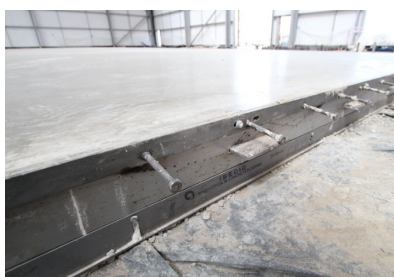
(a) Construction joint
