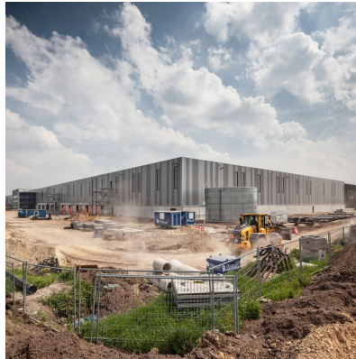
Figure 1.1: Distribution centre under construction [2]
