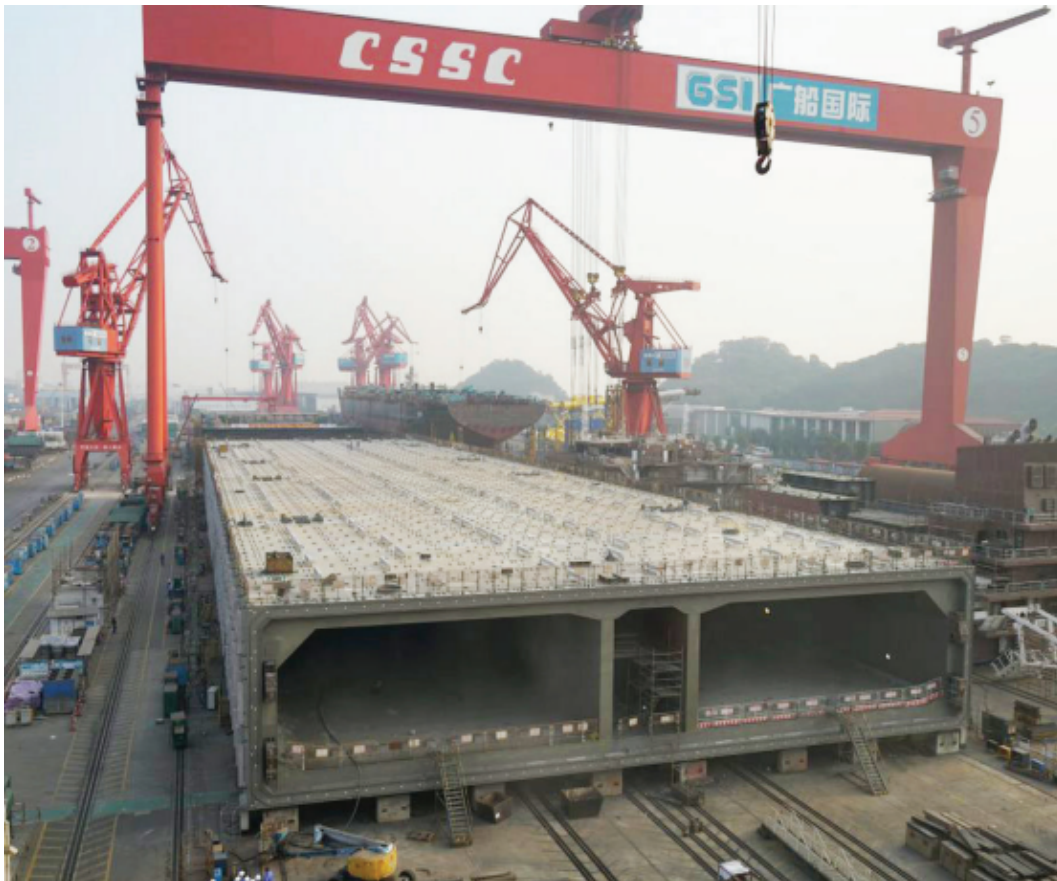
Figure 3.1: Cross-section of Shen-Zhong Tunnel [13]
