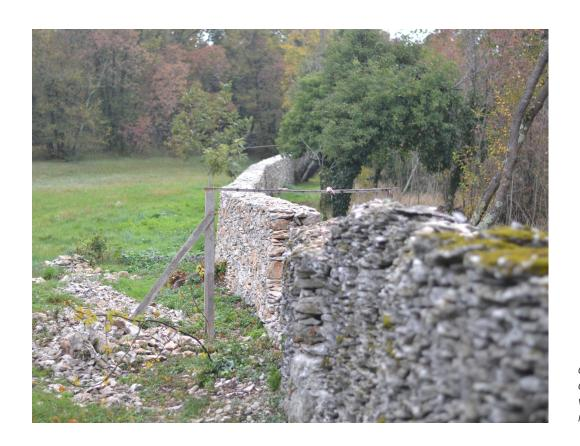
dry stone wall under construction, using a wooden construction for reference
