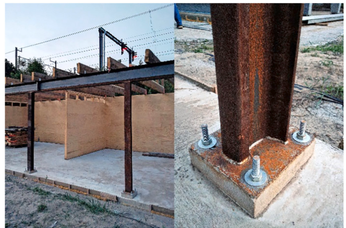
Photo 4. Circular re-use of materials and a symbolic reference to the cultural history of WSK at HvC: railway-tracks as columns of the pavilions, as seen during construction in 2017.
