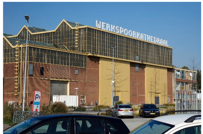
Photo 1. The redeveloped Werkspoor-kathedraal in 2018.
