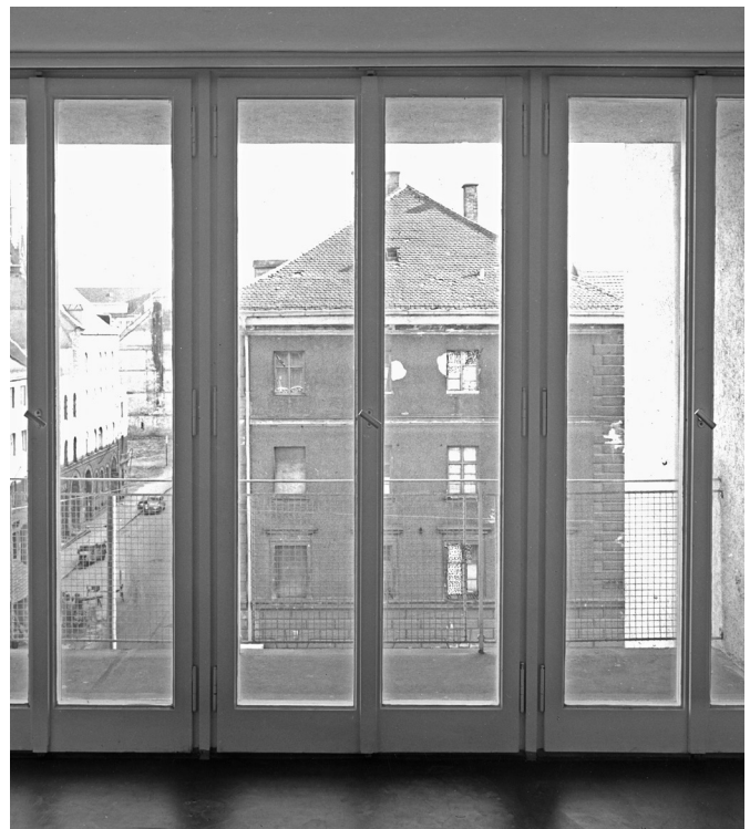
Figure 11: Image of the lintel-less windows
