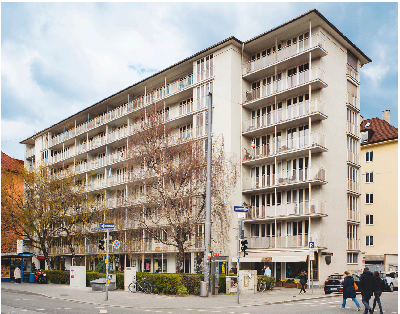
Figure 15: Apartment building Theresienstraße 46-48 today
