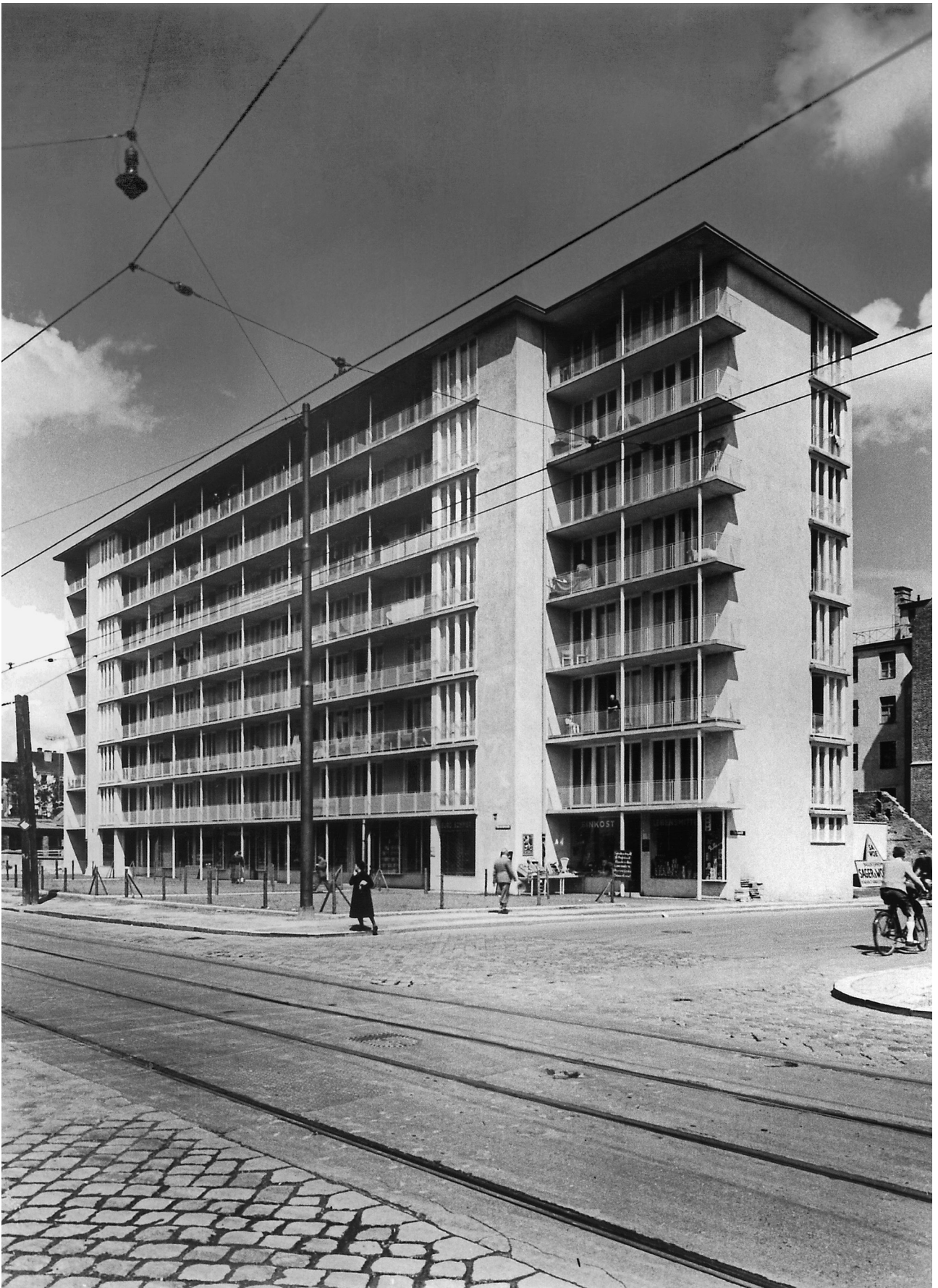
Figure 5: Image of the Theresienstraße apartment building
