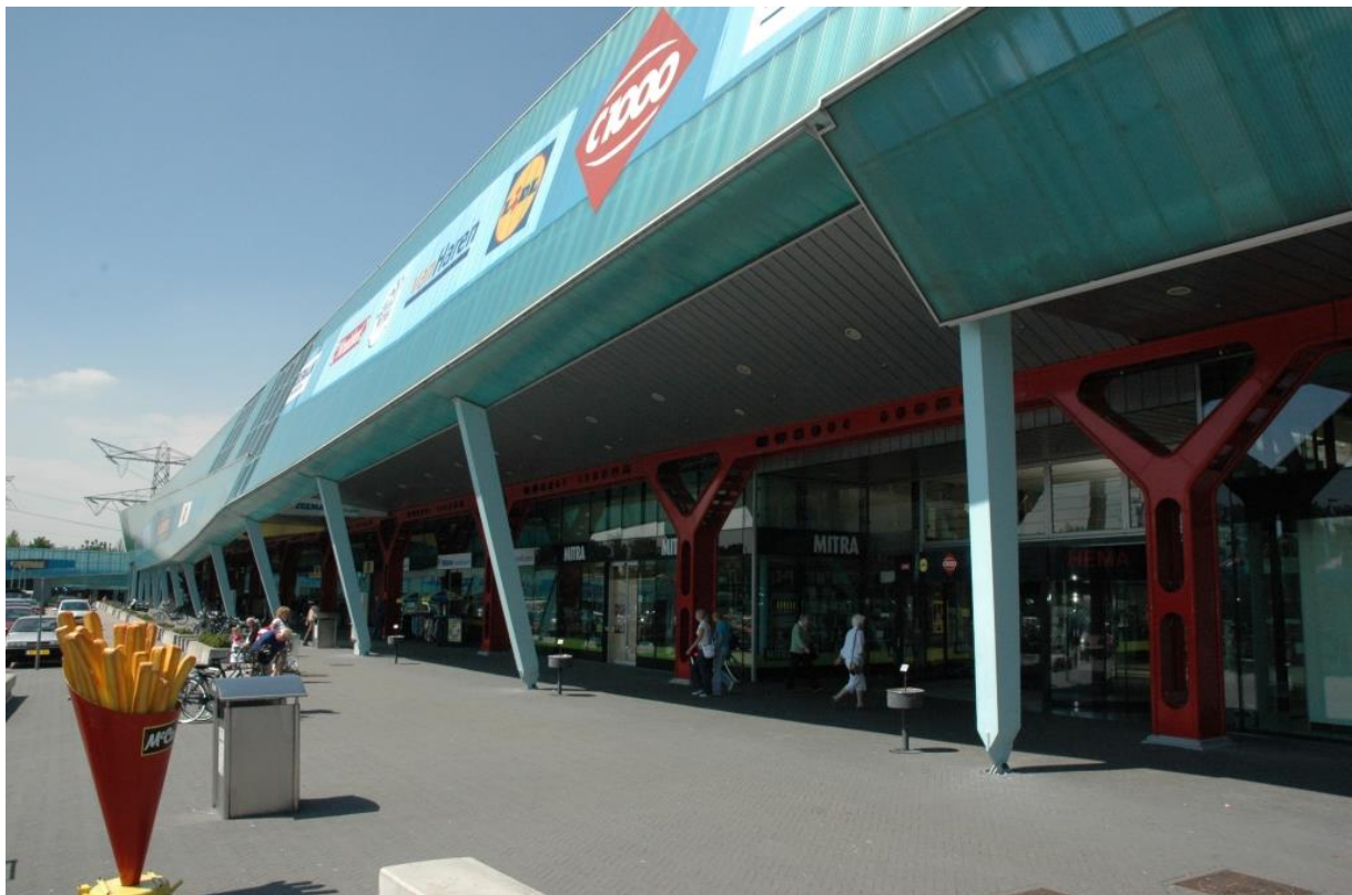
Closer view of the construction ( http://www.rodeca.de/?L=1 )
