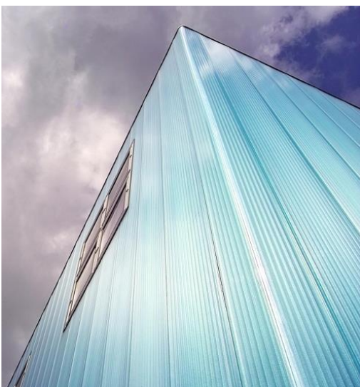
Continuous surface of the corner ( https://kluedo.ub.uni-kl.de/home )
