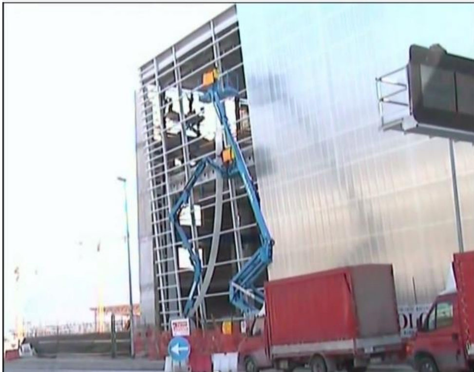
Panel installation by Rodeca ( http://www.rodeca.de/?L=1 )
