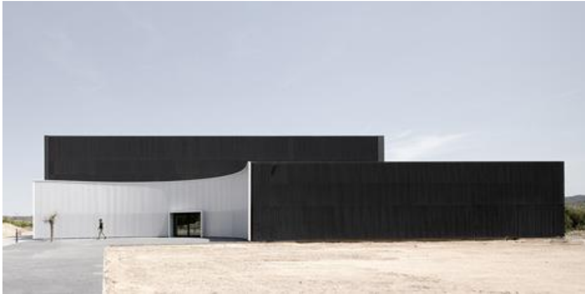
Elevation view of the museum with the curved surface of polycarbonates ( http://www.dezeen.com/ )
