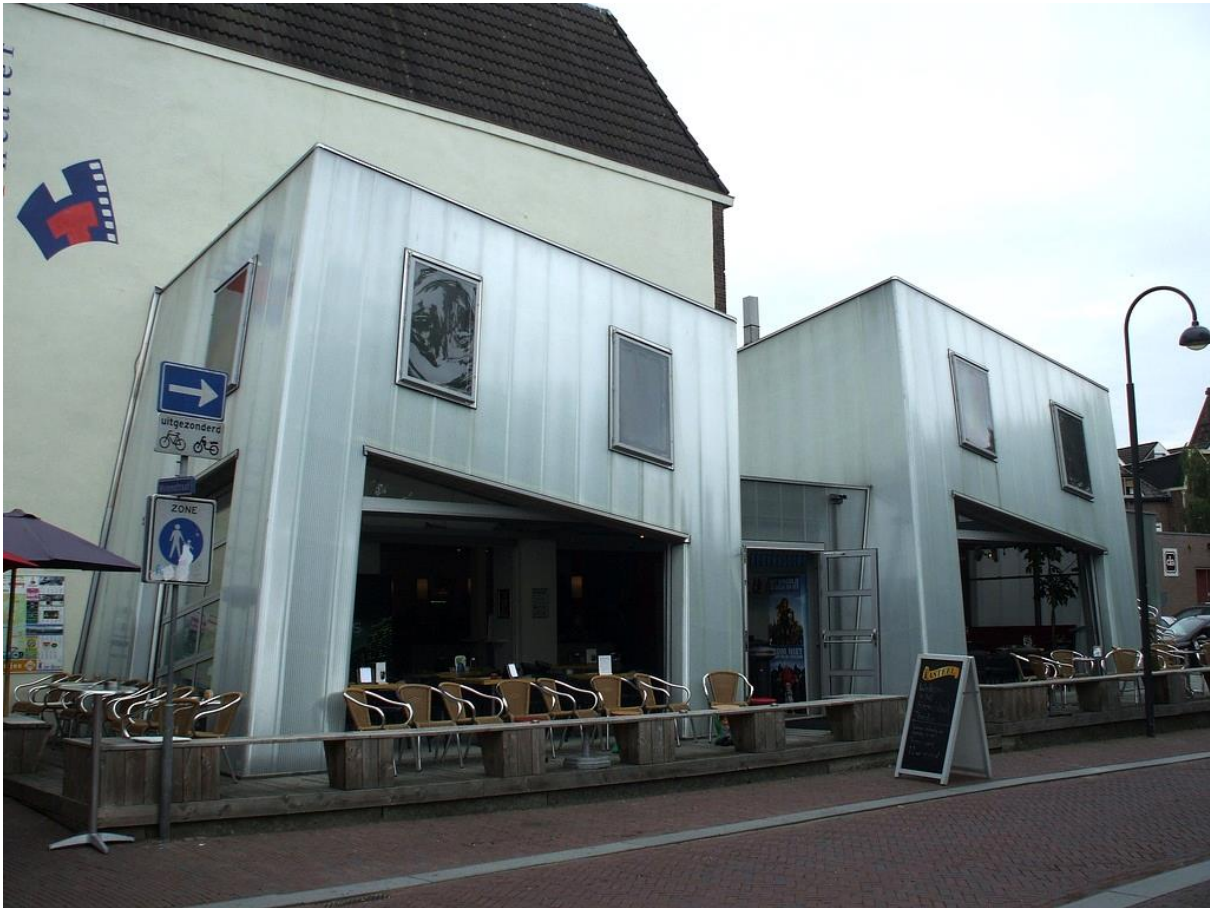
The two volumes are under an angle and special profiles were used to support the facade panels ( http://www.ontwerpburo-roza.nl/ )
