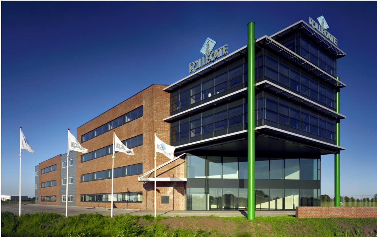
Closer image of the building with the glass facade
