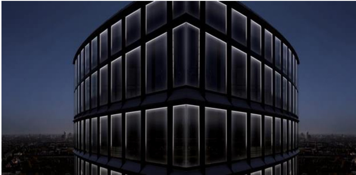
Night impression of a building illuminated by the Lightskin (Shuco Lightskin manual)
