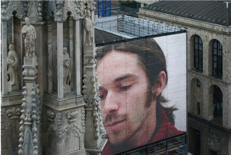
Media mesh facade using 50 x 50 mm pixel pitch in Italy by GKD ( http://www.gkdmediamesh.com/applications/mediamesh.html )
