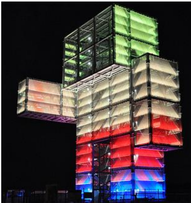
Indemann features a transparent façade made of Illumesh® stainless steel metal fabric with interwoven LED profiles ( http://www.gkdmetalfabrics.com )
