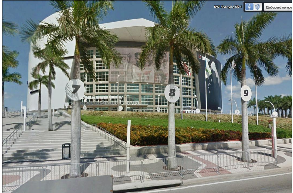
Miami American Airlines Arena (6000 nits) west facade 50 mm pixel pitch from 70 m viewing distance-direct sunlight
