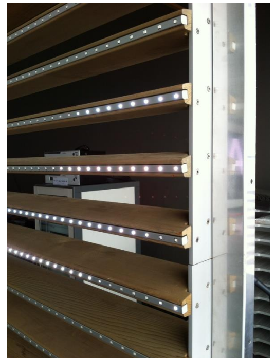
VML technologies with aluminium and timber louvers including LED lights on the front edge (Rollecate)
