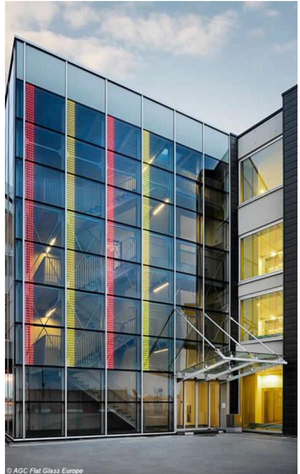
Brussels Airport facade in the afternoon with the project by AGC ( http://www.glassonweb.com/ )
