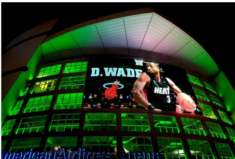
Media mesh facade using 50 x 50 mm pixel pitch in Miami by GKD view by 20 m ( http://www.gkdmediamesh.com/applications/mediamesh.html )
