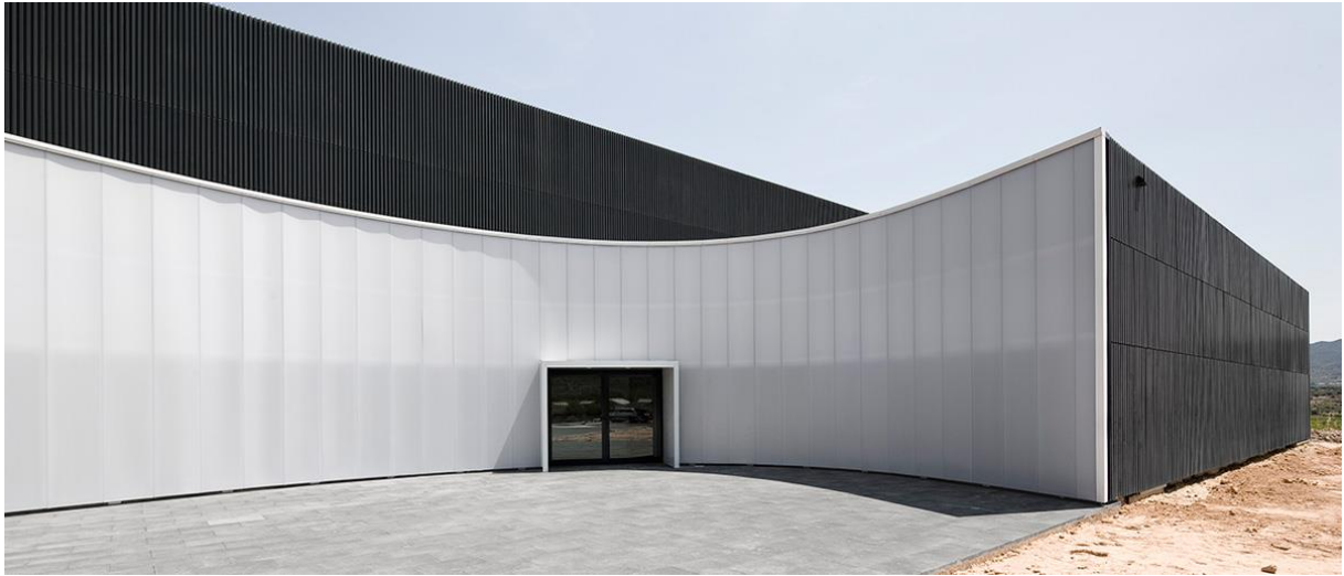
Museum of Energy in Spain with polycarbonate facade ( http://www.archiscene.net/ )
