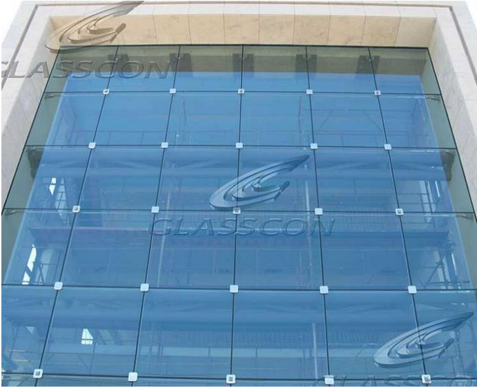
Office building in Athens using 2D inox system ( http://www.glasscon.com/ )
