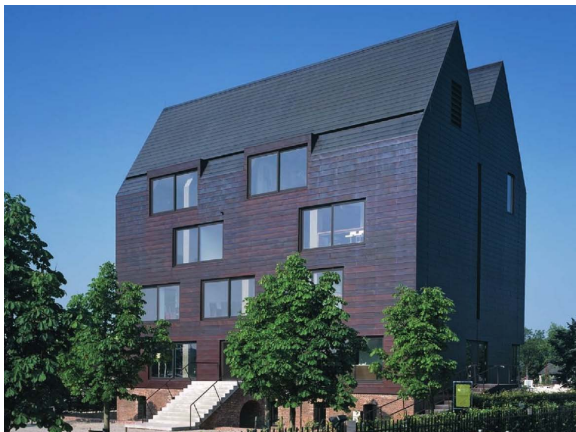
Figure 1.3 House de Wiers Five storey heavy timber frame building Source: JDdV Architecten
