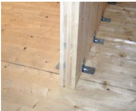
Figure 3.16 Platform frame method Source: Trada
