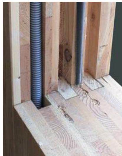
Figure 3.10 Services within panel Source: Binderholz
