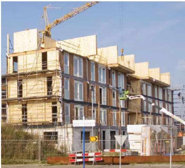
Figure 3.3 Massive timber structure Source: Buro Tichelaar
