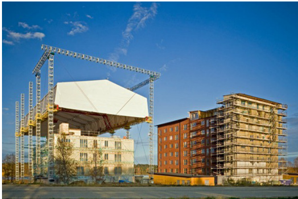
Figure 4.14 Tent with overhead crane Source: Växjö University
