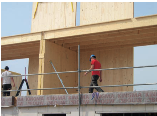
Figure 4.8 Floors discontinuous walls Source: Houtwereld 2007 - 06
