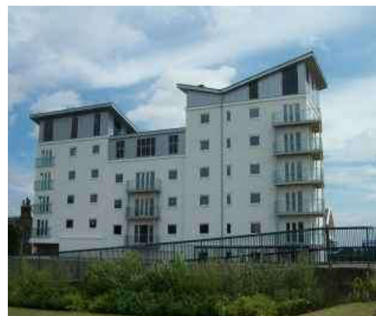
Figure 1.2 St. James Building Six storey light weight timber frame building Source: Trada
