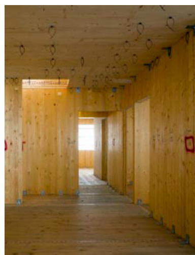
Figure 4.35 Easy fixing of services to ceiling Source: Trada
