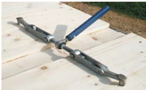
Figure 3.14 Securing of floor panels Source: Binderholz
