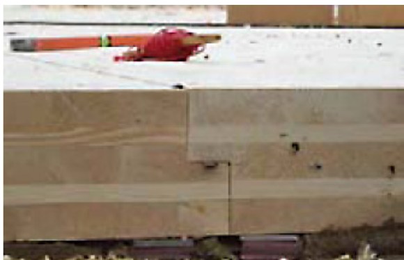
Figure 3.13 Half-lapped joint Source: Trada WIS 2/3-61
