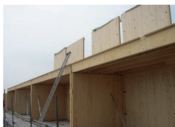
Figure 4.9 Continuous stabilizing walls Source: Houtwereld 2007 - 06
