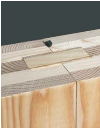
Figure 3.9 Wall connection with jointing piece, Source: Binderholz
