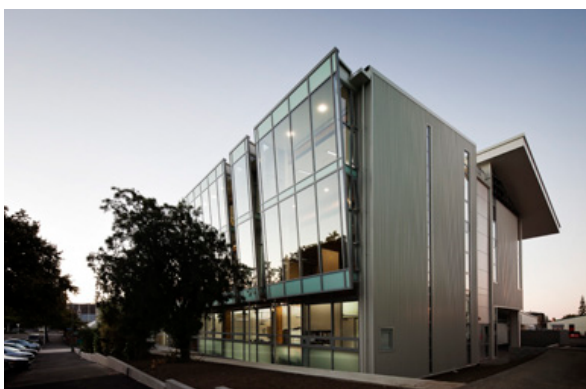
Figure 1.5 NMIT Arts and Media Building Three storey post-tensioned timber frame building Source: Irving Smith Jack Architects
