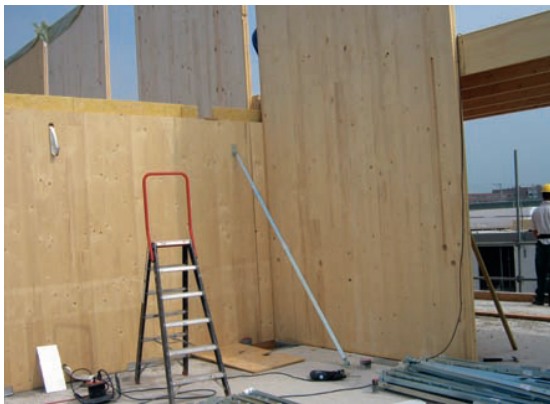
Figure 4.6 Continuous stabilizing walls Source: Houtwereld 2007 - 06
