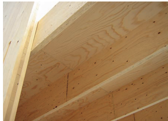
Figure 4.7 Joint sensitive to flanking sound Source: Houtwereld 2007 - 06
