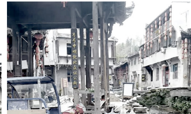
Scenic area renovation activities disturb residents' normal life
