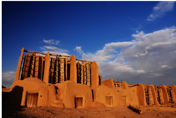
Figure 2.3: Persian vertical axis windmills, primarily used for grist milling and in the sugarcane industry. 1
