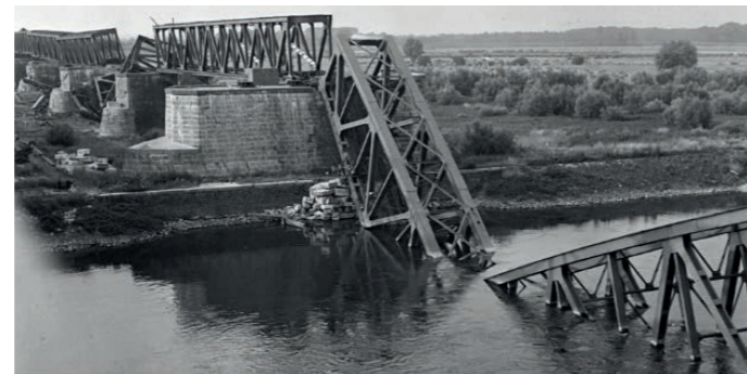
Figure 118: Collapsed bridge during the Second World War (Mom & Filarski, 2008)
