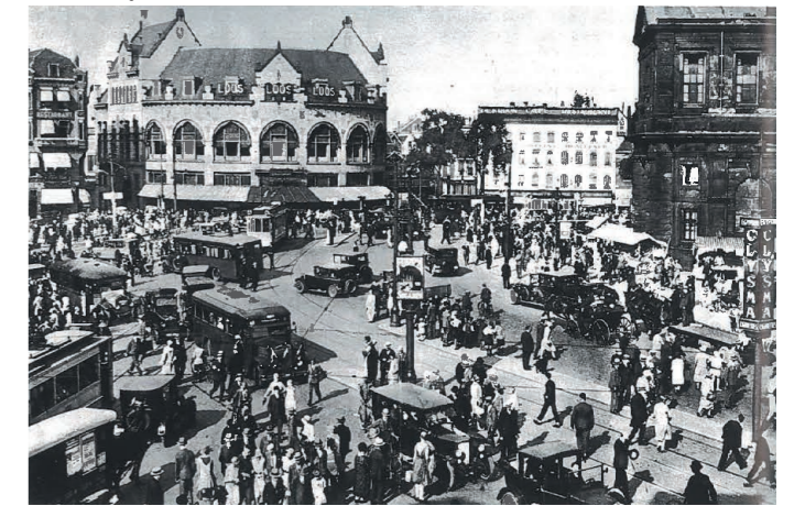
Figure 116: City traffic at the end of the 1920s at Hofplein in Rotterdam (Mom & Filarski, 2008)
