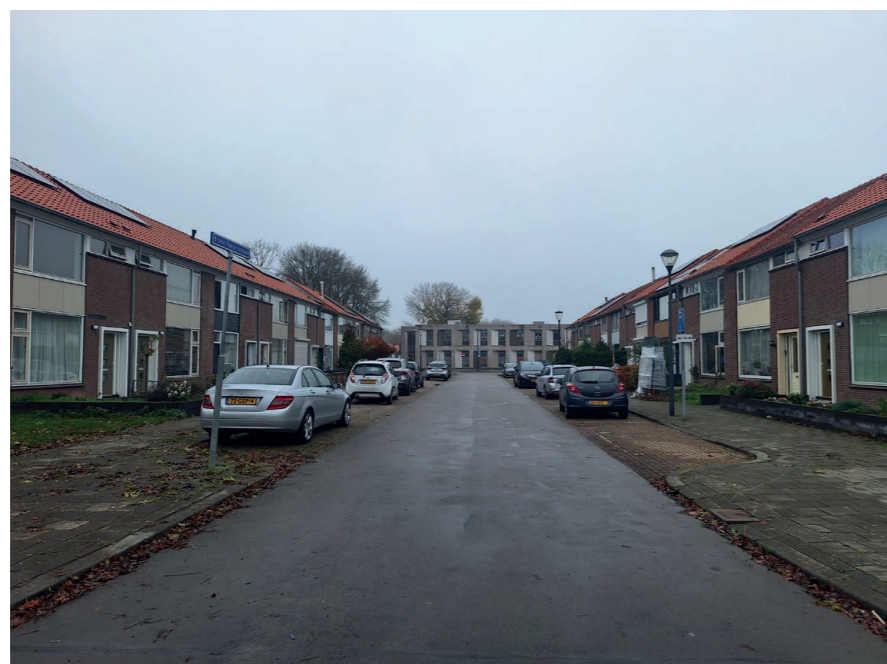
Figure 100: Typical residential street in Hoge Vucht
