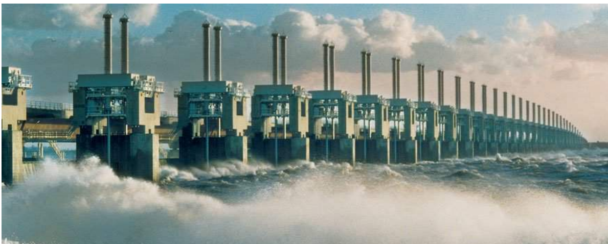
Figure 1.1: The Eastern Scheldt storm surge barrier. Reprinted from Deltapark Neeltje Jans , n.d., Retrieved August 28, 2018, from https://www.neeltjelijans.nl/deltawerken .
