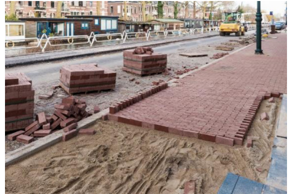
Figure 2.15. Brickstone replacement on pavements 9
