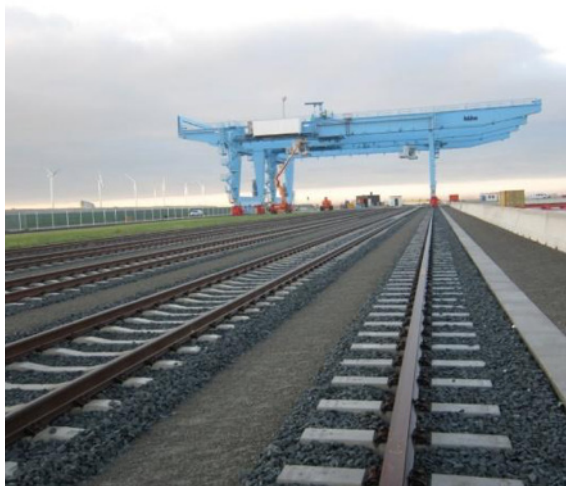
Figure 2.16. Track ballast on railways 10
