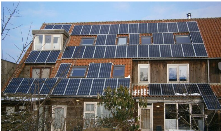
Figure 1-2 Non-integration of PV panels on the roof
