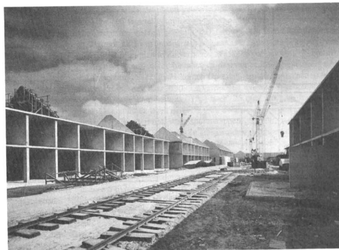
Figure 2-7 Typical building site in the Netherlands with cranes on the rails (Thijssen, 1999)
