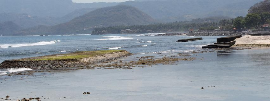
Figure E-3: Breakwaters at Candidasa beach. Own Figure.
