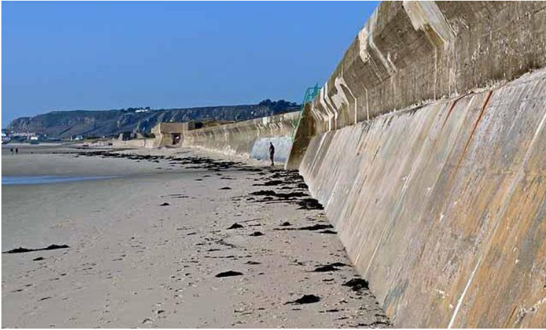
Figure E-2: Seawall at La Crabiere (Dixon, 2011).
