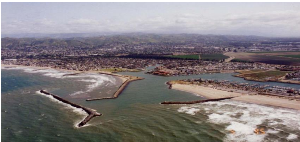
Figure E-7 Jetties and Navigational Breakwater at Ventura Harbour (USACE, 2012).
