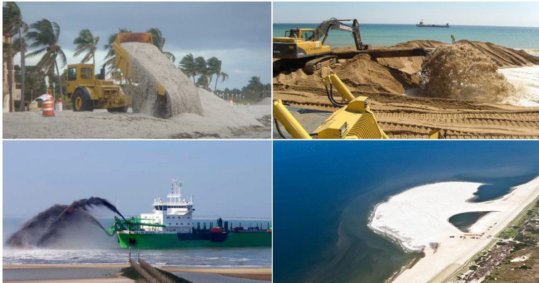
Figure E-9: Methods for beach nourishment, clockwise starting top left: Conventional filling (Hollywood Margaritaville, 2015). Pumping sand from dredge vessel (URBANE, 2015). Sand motor in the Netherlands (van Houdt, 2011). Rainbowing from dredge vessel (Climate Tech, 2015).
