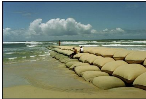
Figure E-11: Geo-textile Sand Containers (ElcoRock, 2015)
