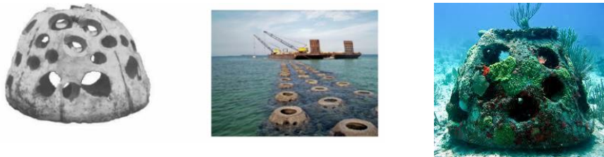
Figure E-13: Reef Ball and Reef Ball implementation (Bargado, 2013).
