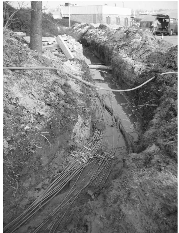
Fig. 1. Trench with dozens of cables.
