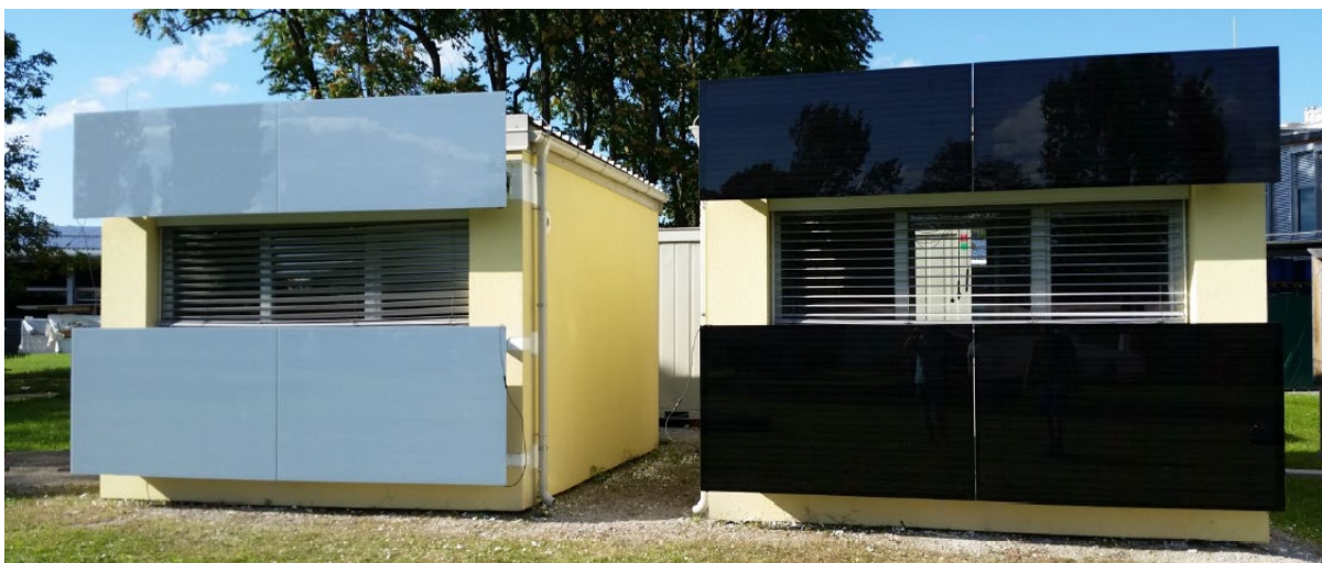
Figure 2.6 'COOLSKIN' testing facade
