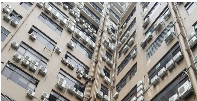
Figure 1.19 An air-conditioning city
