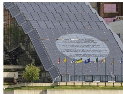
Roof with BIPV
