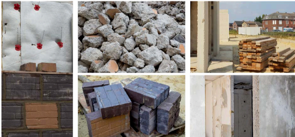
Figure 4.11. Construction technique 2: Reuse by remanufacturing (R6 following Potting et al., 2017). On the left reused insulation from the flat (top) and brick modules (bottom left and middle) as used in Type B. Top middle is the crushed concrete as used in Type A. On the right the wooden door frames (top) which have been reused and the partitioning walls (bottom) (Durmisevic, 2019b).
