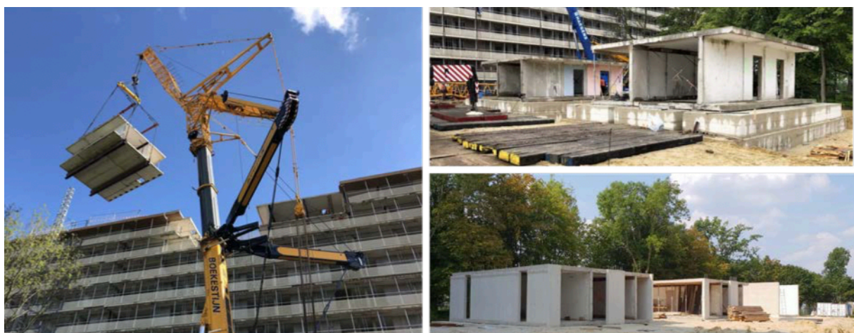
Figure 4.10. Circular construction technique 1: Direct reuse (R4 following Potting et al., 2017). Used for Type A and B (Durmisevic, 2019b).
