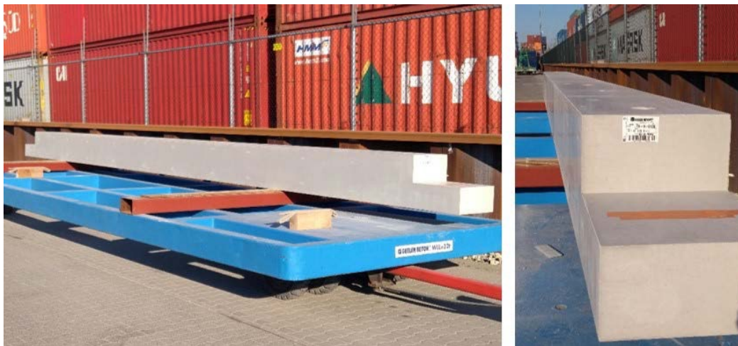
Figure 4.18. Modular load bearing circular concrete system, the concrete aggregate is supplied by the deconstruction company, developed by prefab concrete supplier and assembled by the construction company. Picture derived from Durmisevic (2021).
