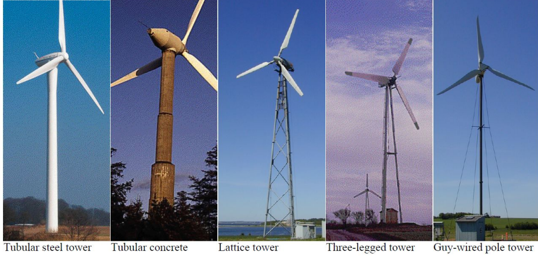
Figure 5.3: Wind turbine tower types [44].
