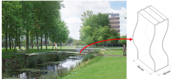
Figure 1 Aspect of the Glass Masonry Bridge and the brick shape
