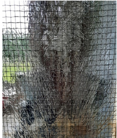
Hand-made wired glass in the Van Ravesteyn House, Utrecht (1932). Evidence of a corrugated roller pushing the wire net in the viscous glass can be seen on the surface of the panel as body marks (wrinkles).
