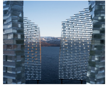
Unesco cast glass pavilion in Sarfannguit, Greenland, in progress (2021). Designed by Konstantin Ikonomidis. Glass Engineering by TU Delft Glass Lab. Image by Julien Lanoo.
