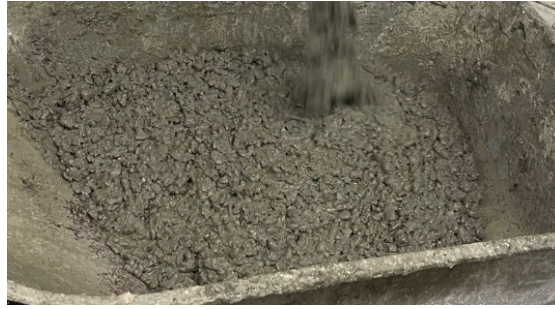
Figure 7.10: Visual inspection of the consistency of fresh concrete
