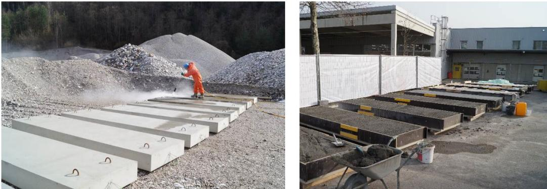
Figure 3.3: Surface treatment and concreting at construction yard [4]
