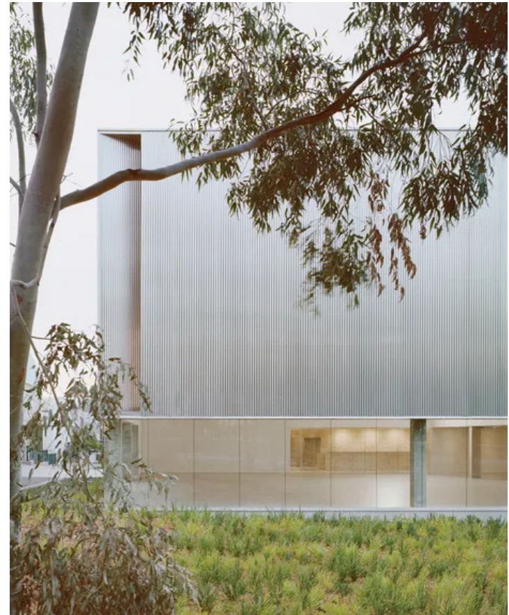
Lahznimmo Architects, museum discovery centre
