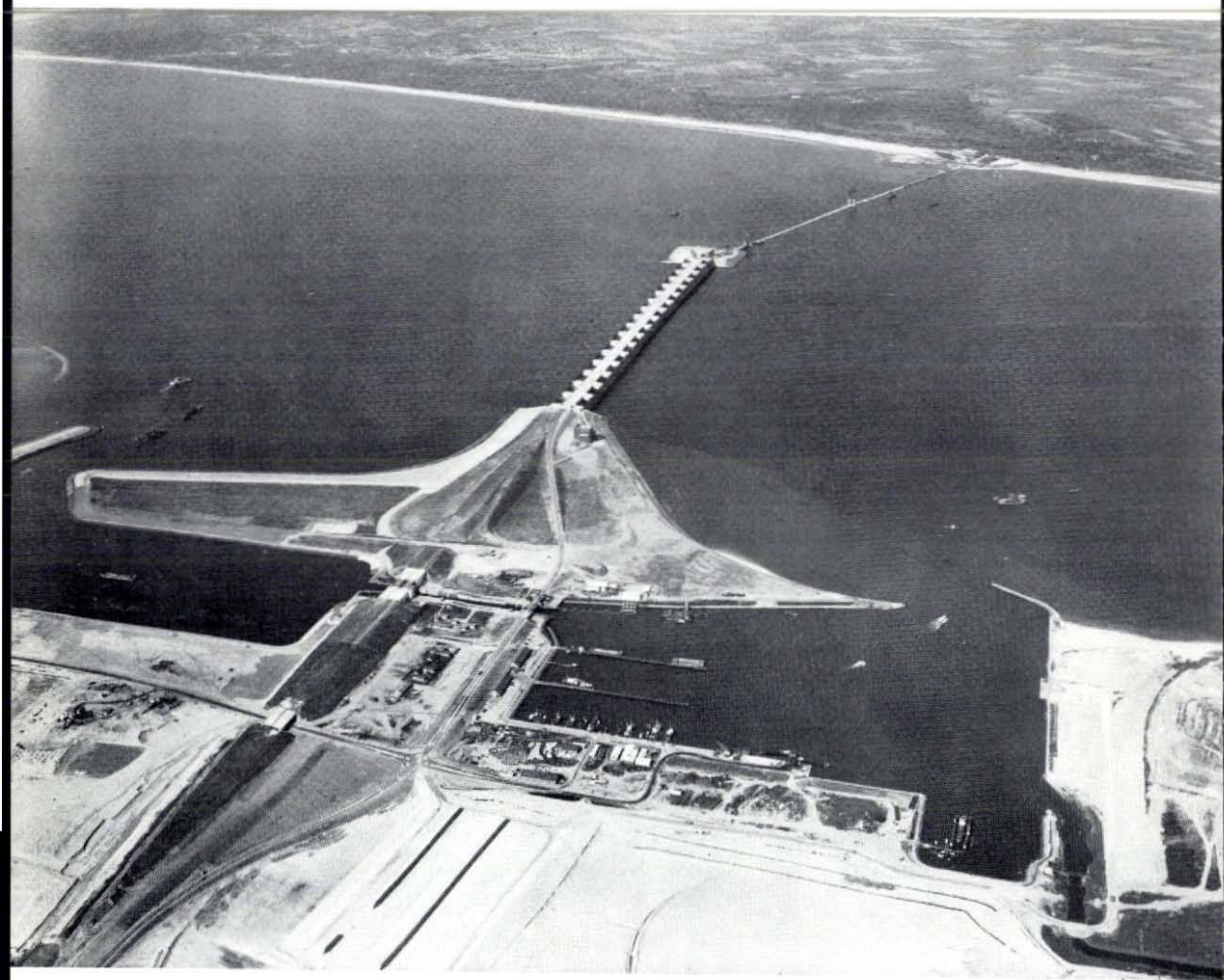
Photograph 3. General view of the sluice-gate complex in the closed Haringvliet with the sea on the left. In the foreground the locks for navigation and fishery (photo Bart Hofmeester)
