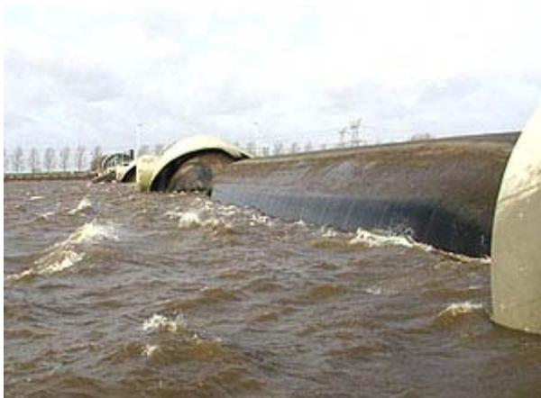
**Figure 51:** inflatable barrier near Ramspol (NL).
