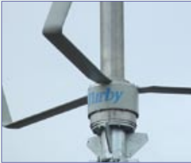
The generator of a Turby is fully integrated in the wind turbine and consists of an external magnetic rotor (the ring bearing the name) that rotates around the stator. The generator does not have any bearings of its own.
