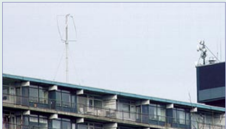
Prototype Turby on the roof of a block of flats in the university town of Tilburg in the south of the Netherlands
