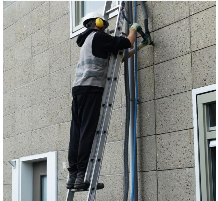
Figure 8: Cleaning, repointing and post-insulating Airey houses in Amersfoort. Photograph: Hielkje Zijlstra
