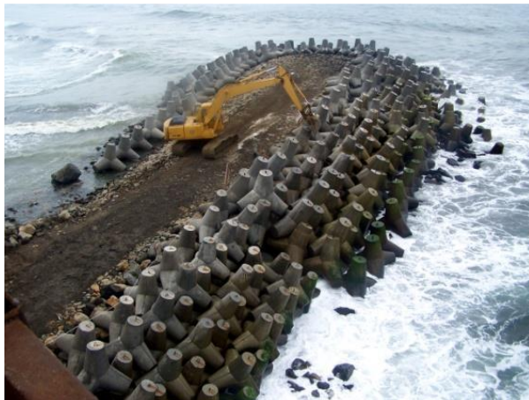
FIGURE 2-4 PLACEMENT OF TETRAPODS
