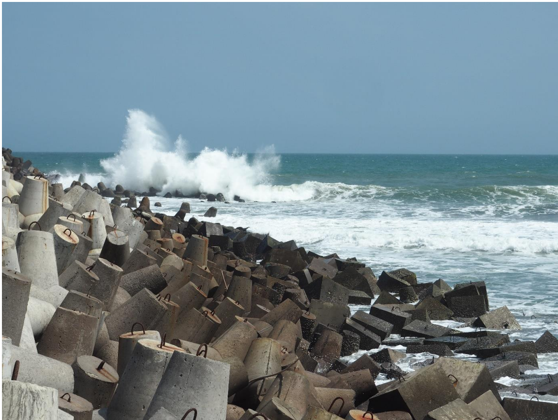
5. The concrete cubes from the toe.
