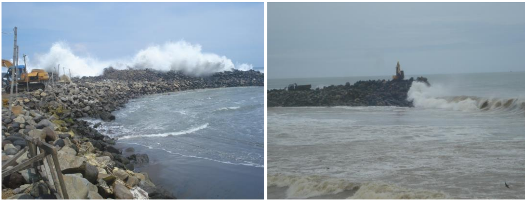
FIGURE H-5 UNSAFE SITUATIONS DURING CONSTRUCTION
