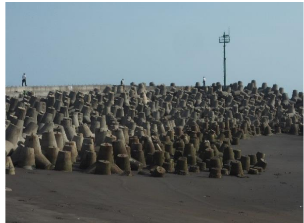
FIGURE 2-5 DISPLACEMENT OF TETRAPODS
