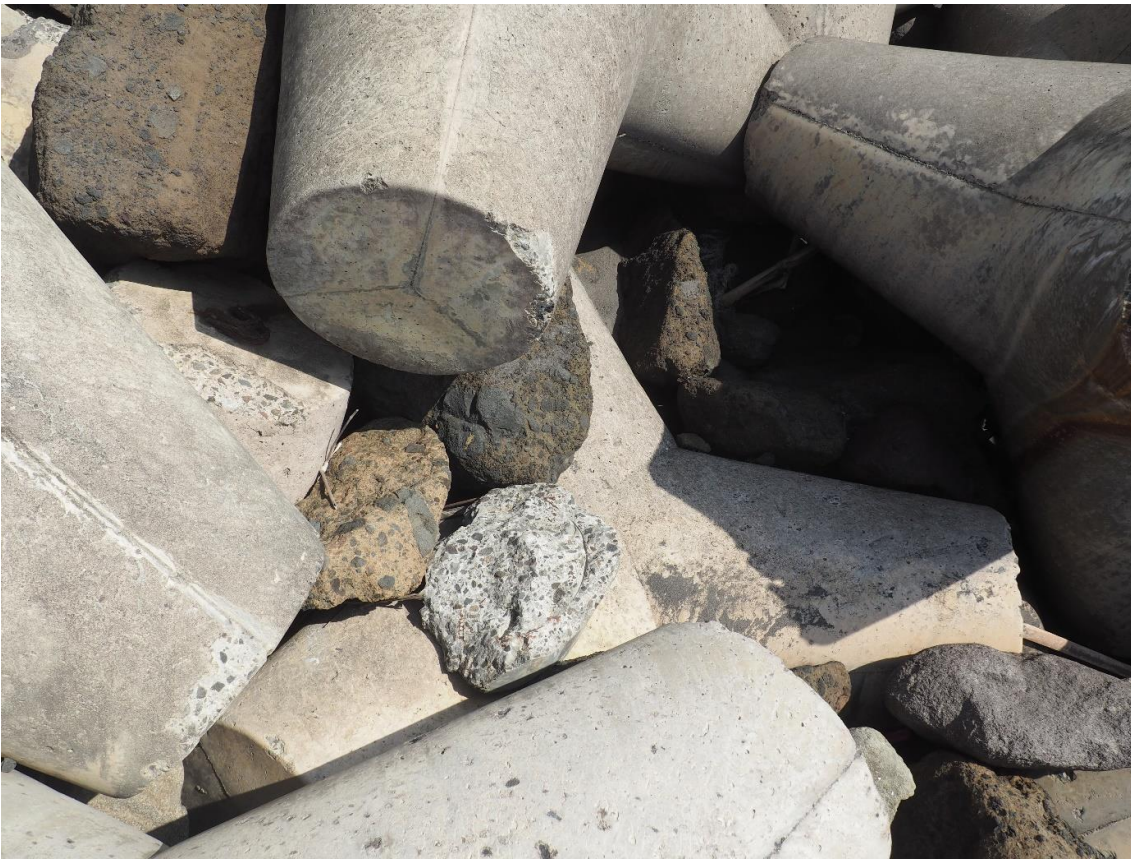
7. At some places there is a double layer tetrapod. This might occur due to collision and slipped off.
