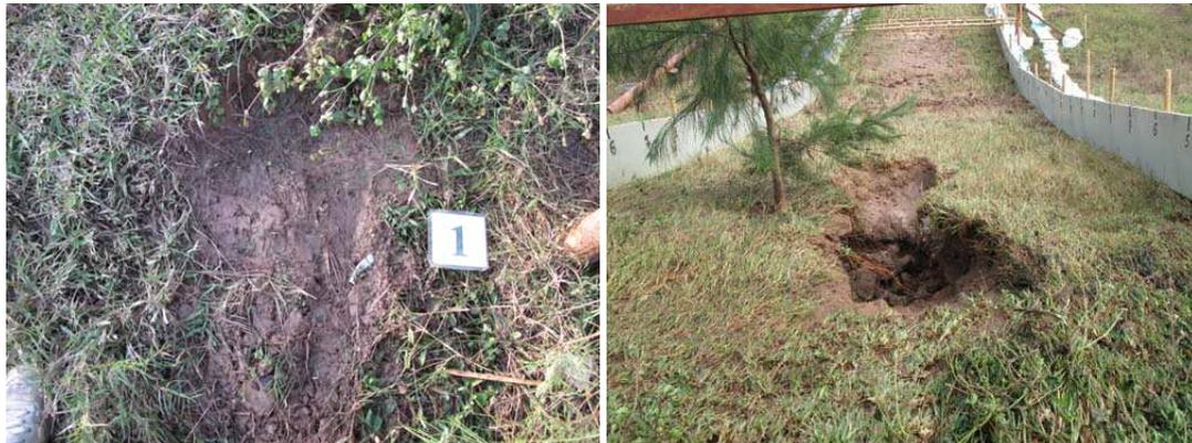
Figure 6. Formation and development of damage on Bermuda grass slope. Left: initial situation. Right: damage was extending to the casuarina root.
