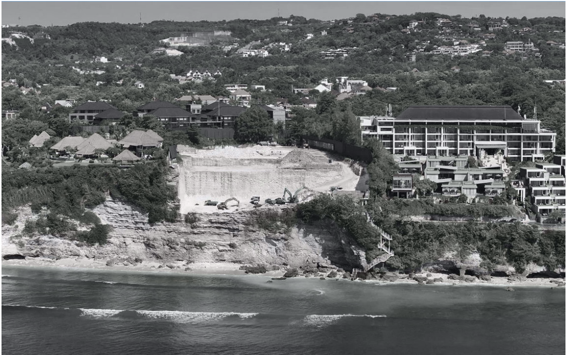
Fig 2.5 Cliff collapse during hotel Construction in Southern part of Bali. Source: Bali Live blog (2024)
