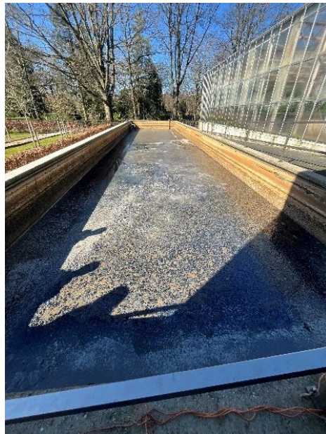
Appendix Figure C.2 MNR Equalization Tank During Overflow 1
