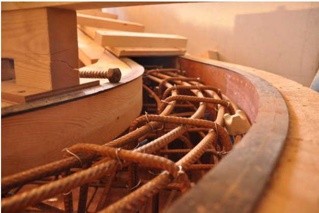
Fig. 1: Complex curved reinforcement under construction at the first phase of the NSP Arnhem.
