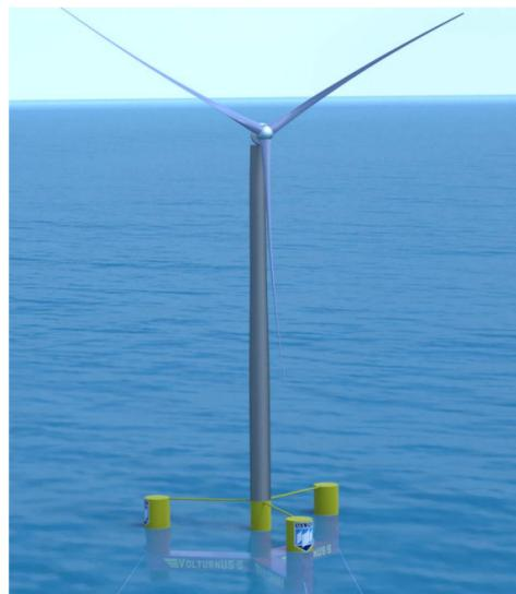
**Figure 4.1:** The UMaine VoltturnUS-S reference semi-submersible platform [25]
