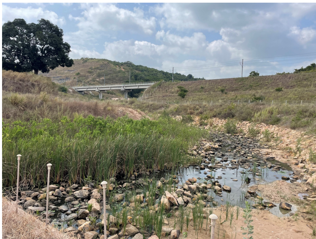
Figure 5.27: SGR near Pugu Hills on 20 February 2025, showing protected riverbanks and an elevated, dam-like structure. A railway viaduct connects the hill on the left to the raised dam-like structure on the right.
