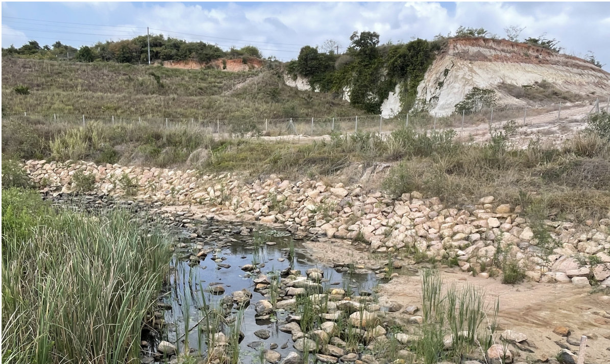
Figure 3.8: Photograph from the February 2025 site visit illustrating the protected and re-vegetated banks in the Upper Basin.
