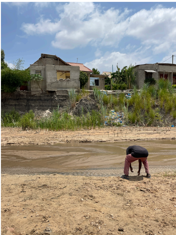
(a) Residential building located on the 5-meter-high riverbank in the Upper Middle Basin, observed during the February 2025 site visit as the first house along the river. Clearly, elevation alone does not guarantee protection from erosion.
