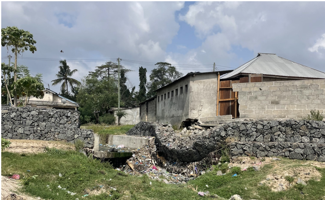
(b) Close-up showing early signs of failure in the installed gabions at the same location.
