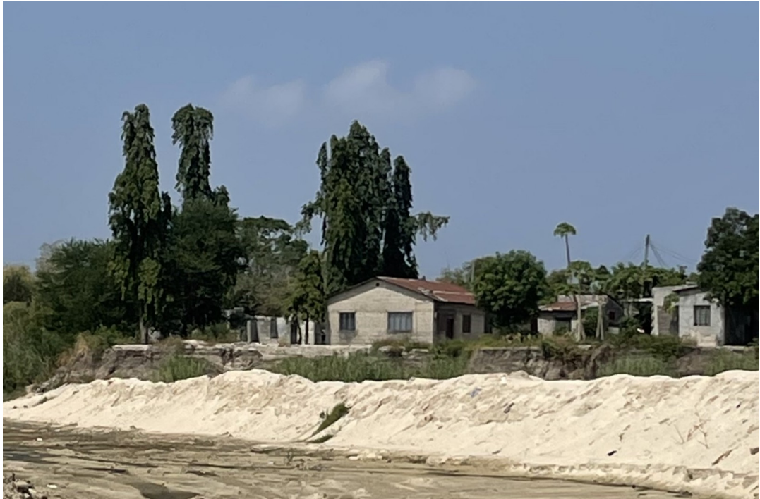
(b) Photo taken in the Upper Middle Basin at the exact location shown in figure 6.7a, during a field visit. The image shows the southern bank, where houses are located close to a steep riverbank. A manually constructed reinforcement is visible in the foreground, built out of loose white sand to protect against erosion.
