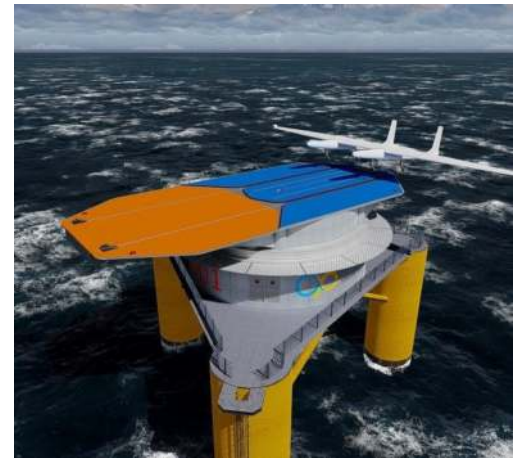
Impression of offshore floating airborne wind energy system.
