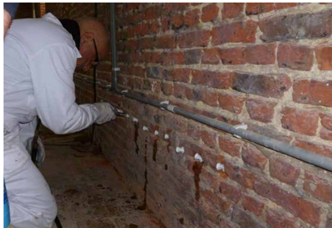
FIG. 3.5 Injection of a liquid product by means of pressure / Photo: B. Lubelli
