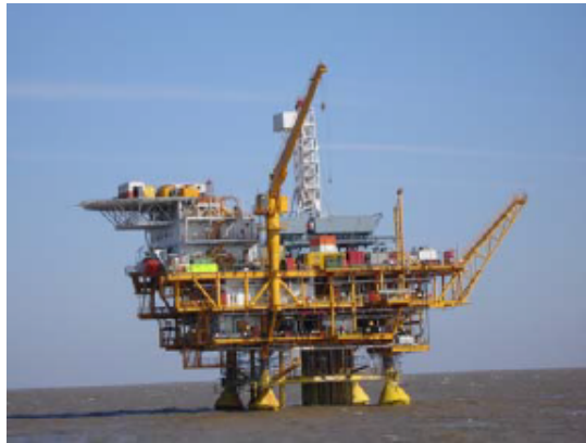
(a) The JZ9-3 WHPA jacket structure.
