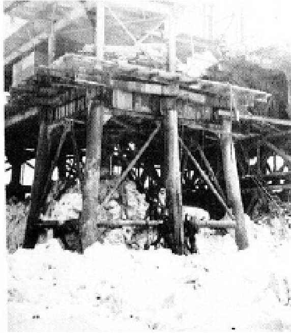
Figure 2.18: The internal ice jam of Bohai No.2, which eventually was pushed over by sea ice. (Xu et al., 2009)
