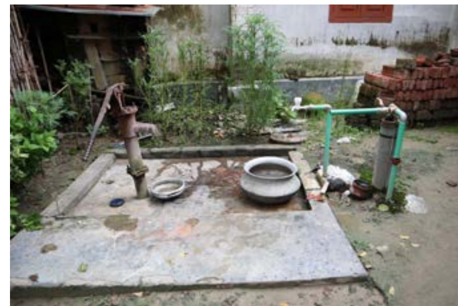
Figure: on the left is your private hand pump, on the right is your tap that is connected to the PWS system.
