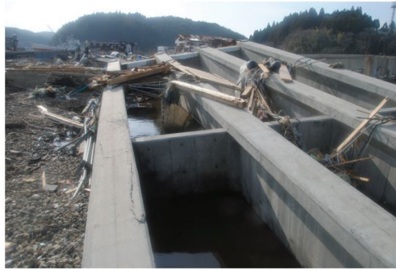
Figure 2.6. Utatsu highway bridge with visible hollow compartments [Kawashima and Matsuzaki, 2012].
