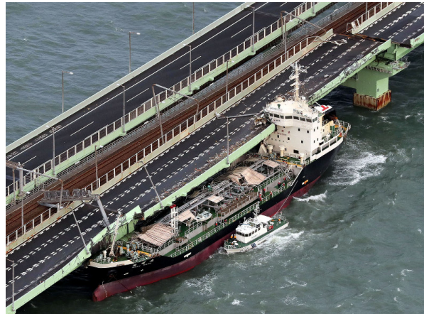
Figure 2.9. Osaka bridge failure due to collision with tanker [Mainichi, 2018].
