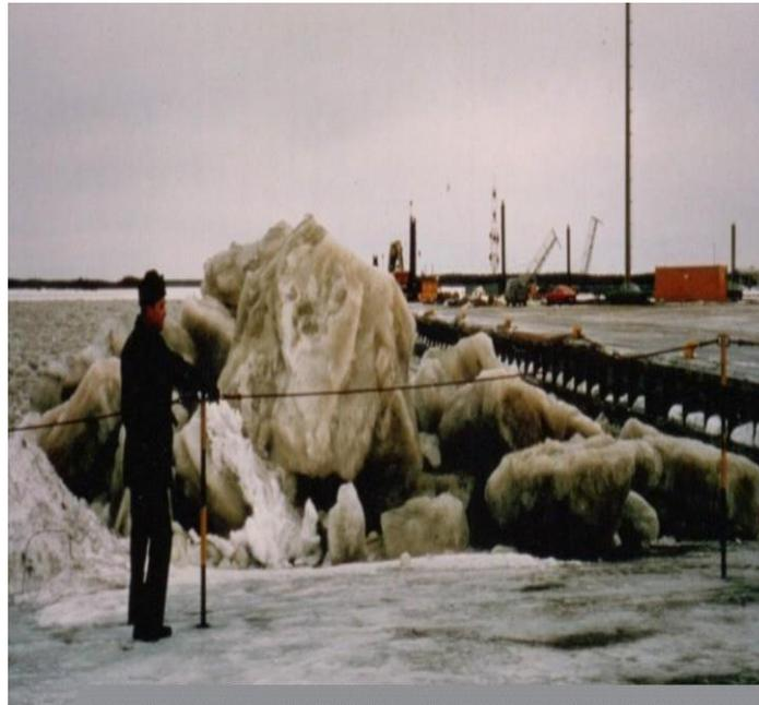
Figure 2-4 Brash ice blocks lifted with cranes from berth area to enable berthing. Ice blocks are glued together by slush in low temperatures forming larger blocks. Extracted from (Saarinen, Suojanen, & Eranti, 2011)
