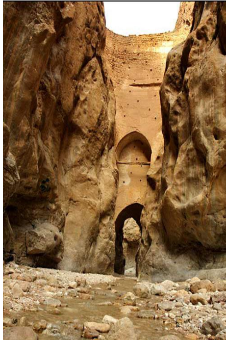
Fig 1. The Abbasi dam 13
