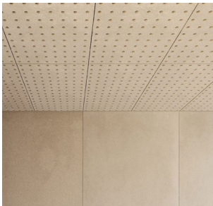
ceiling perforated acoustic panel
