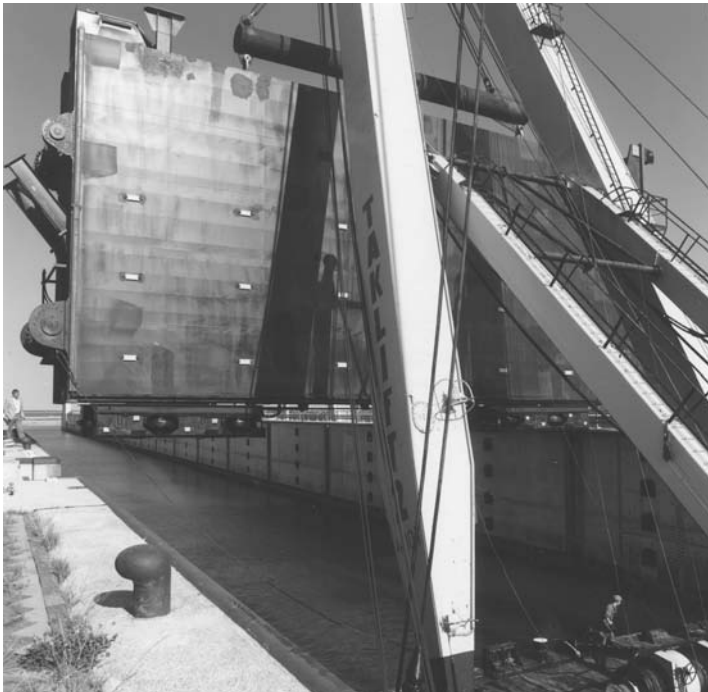
Photo 7.5 Rolling gate at Krammersluizen during installation (1985)
