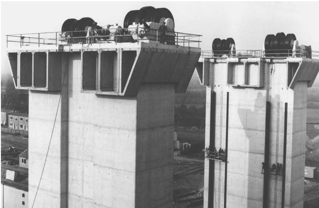
Photo 7.31 Operating mechanism of the lift gate of the new lock in Wijk bij Duurstede
