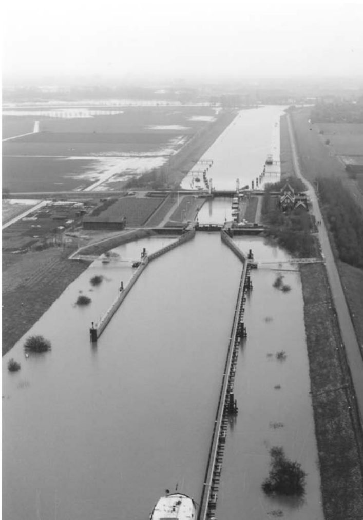
Photo 4.5 Lock approaches at the lock at Engelen
