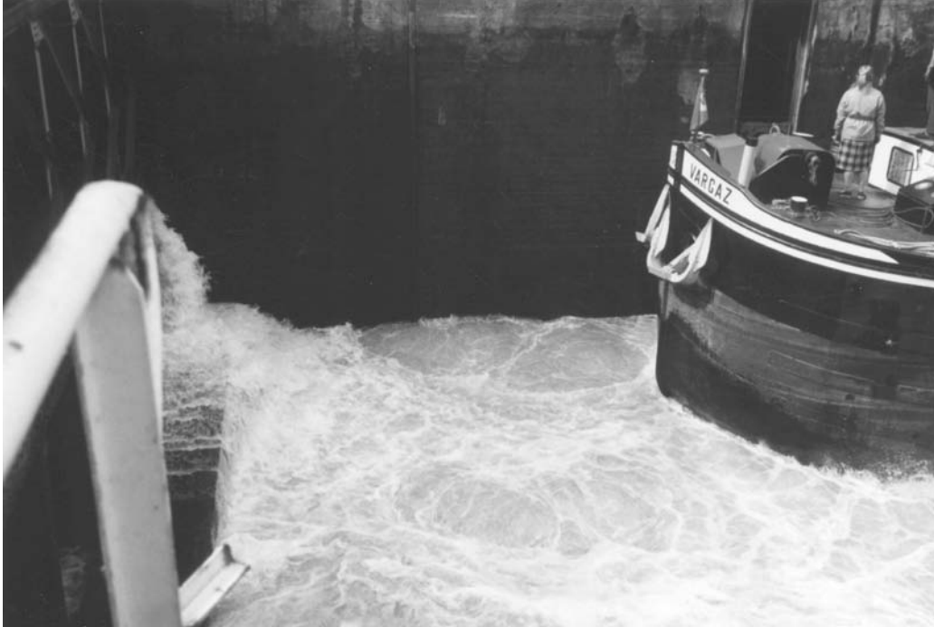
Photo 6.2 Flow pattern during filling by means of lifting the upper gate of the old lock in Born
