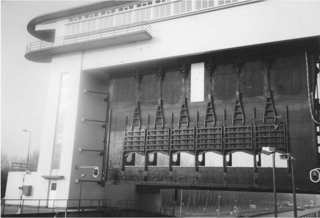
Photo 6.7 Gate openings in the lift gates of the Princess Beatrix locks in Nieuwegein
