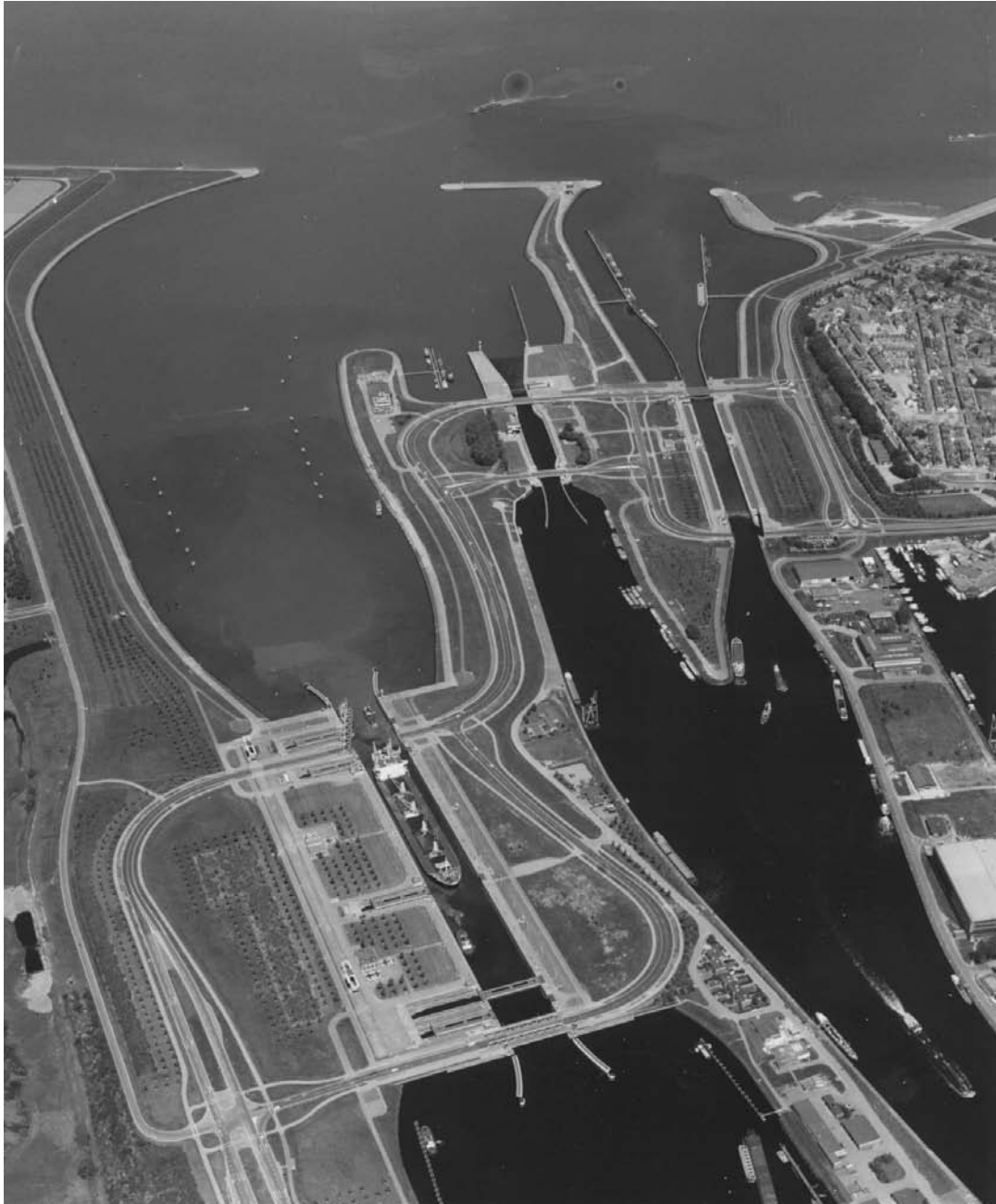
Photo 5.1 Lay out of the lock complex at Terneuzen with (f.l.t.r.) large sea lock, Middensluis and inland navigation lock as link between the Westerschelde (above) with Canal from Gent to Terneuzen (below)
