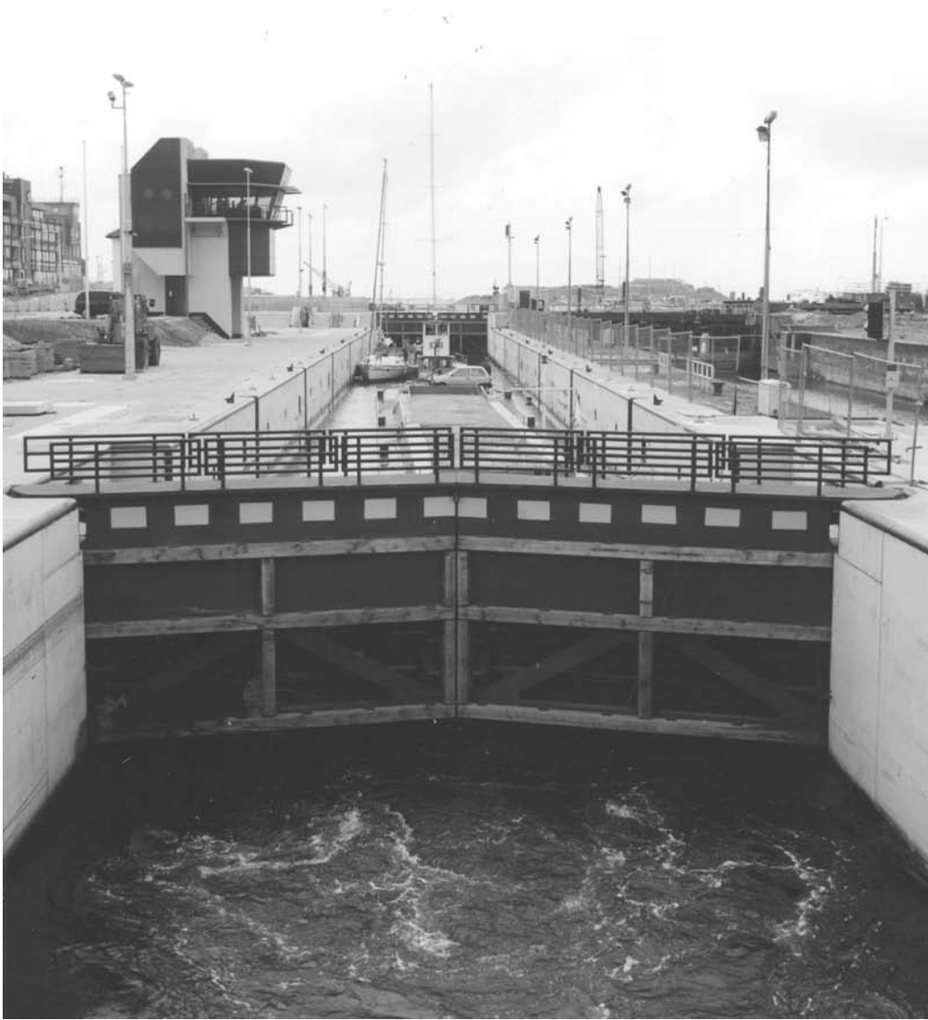
Photo 6.6 Flow pattern during emptying by means of gate openings of Kleine Sluis in IJmuiden
