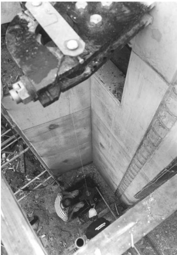
Photo 7.13 Adjusting the pivot of a single pivot gate of the lock in Gorinchem (1987)
