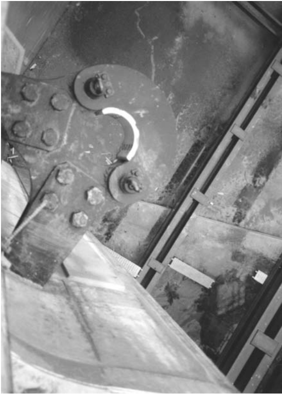
Photo 7.10 Collar of the mitre gate Tweede Sluis in Lith
