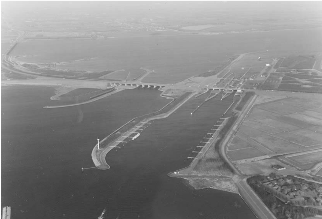
Photo 5.8 Lay out of lock complex Volkerak with (f.l.t.r.) yacht lock, drainage sluice and three push-tow locks as connection of Volkerak (below) with Haringvliet (above)
