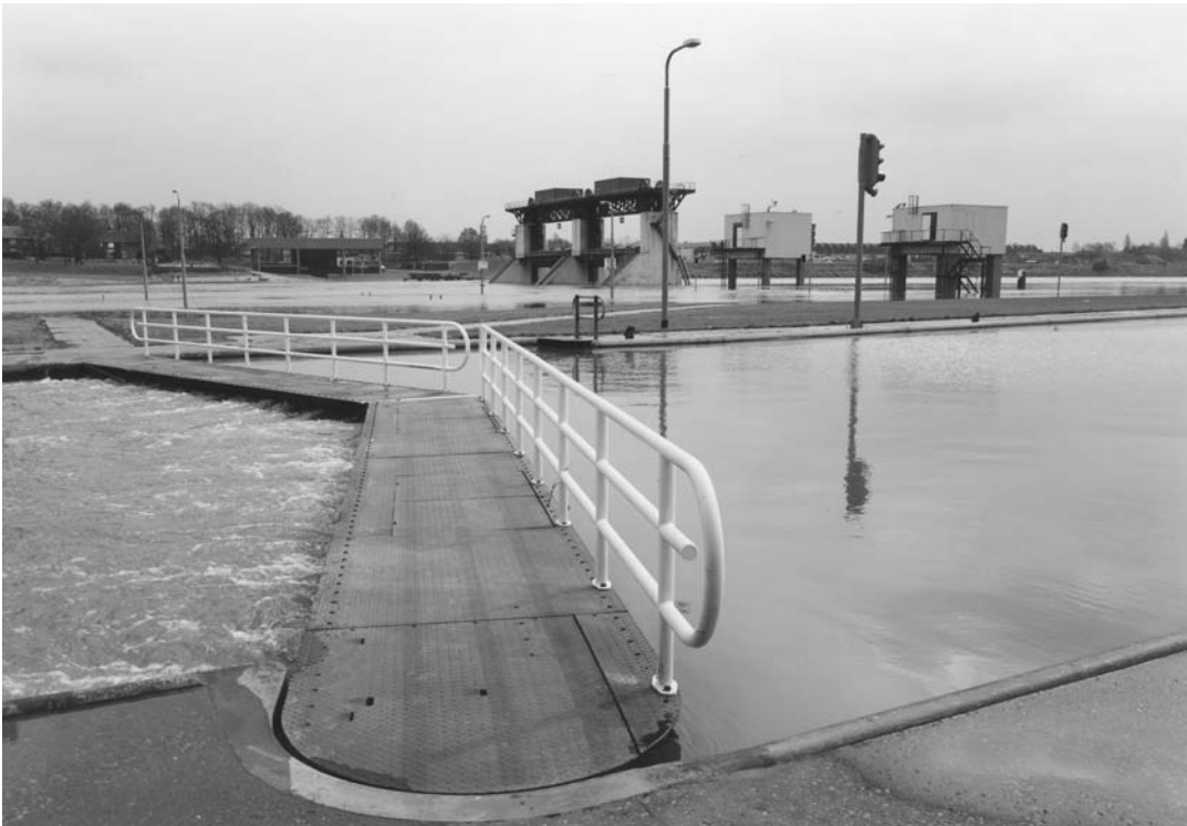
Photo 4.4 High water at weir and lock complex at Belfeld
