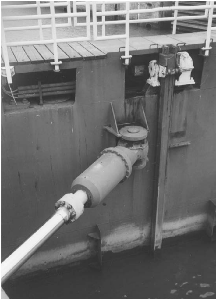
Photo 7.19 Hydraulic cylinder gate operating mechanism and direct rack bar and lock paddle operating mechanism of push-tow locks in the Volkerak
