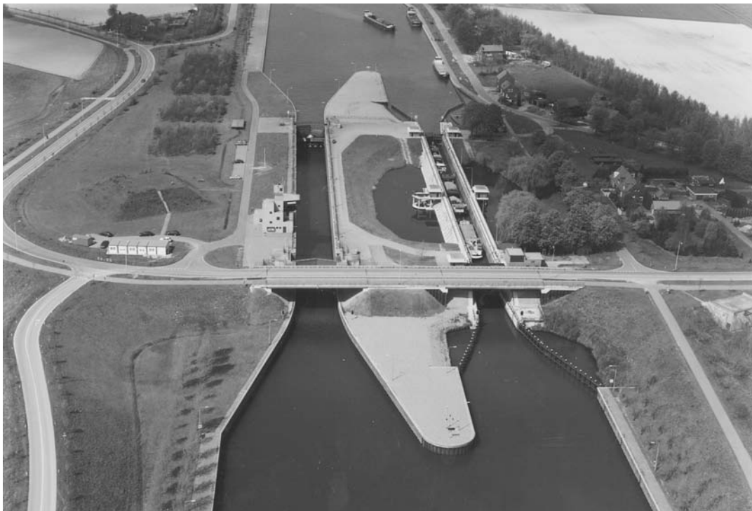
Photo 5.2 Lay out of lock complex at Panheel with new lock with stilling chamber (left) and the old lock with storage reservoirs (right) as connection to the Kanaal Wessem-Nederweert on the Maas
