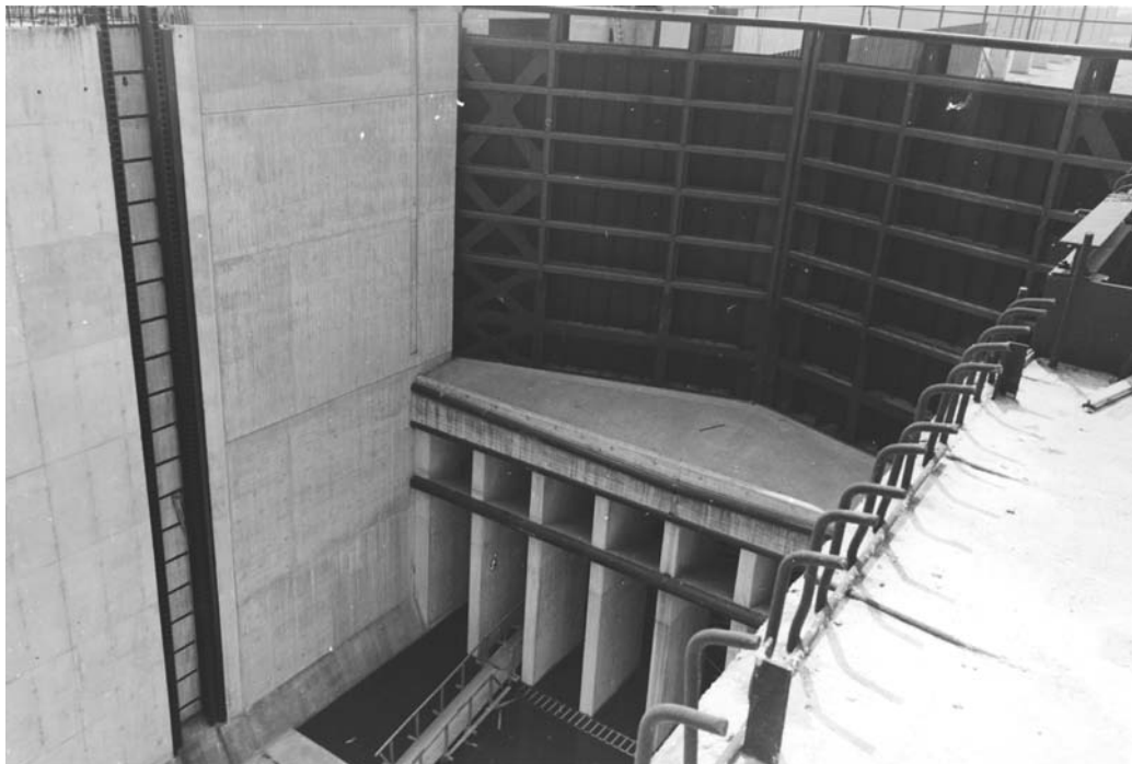
Photo 6.16 Upper head with stilling chamber of locks in Maasbracht
