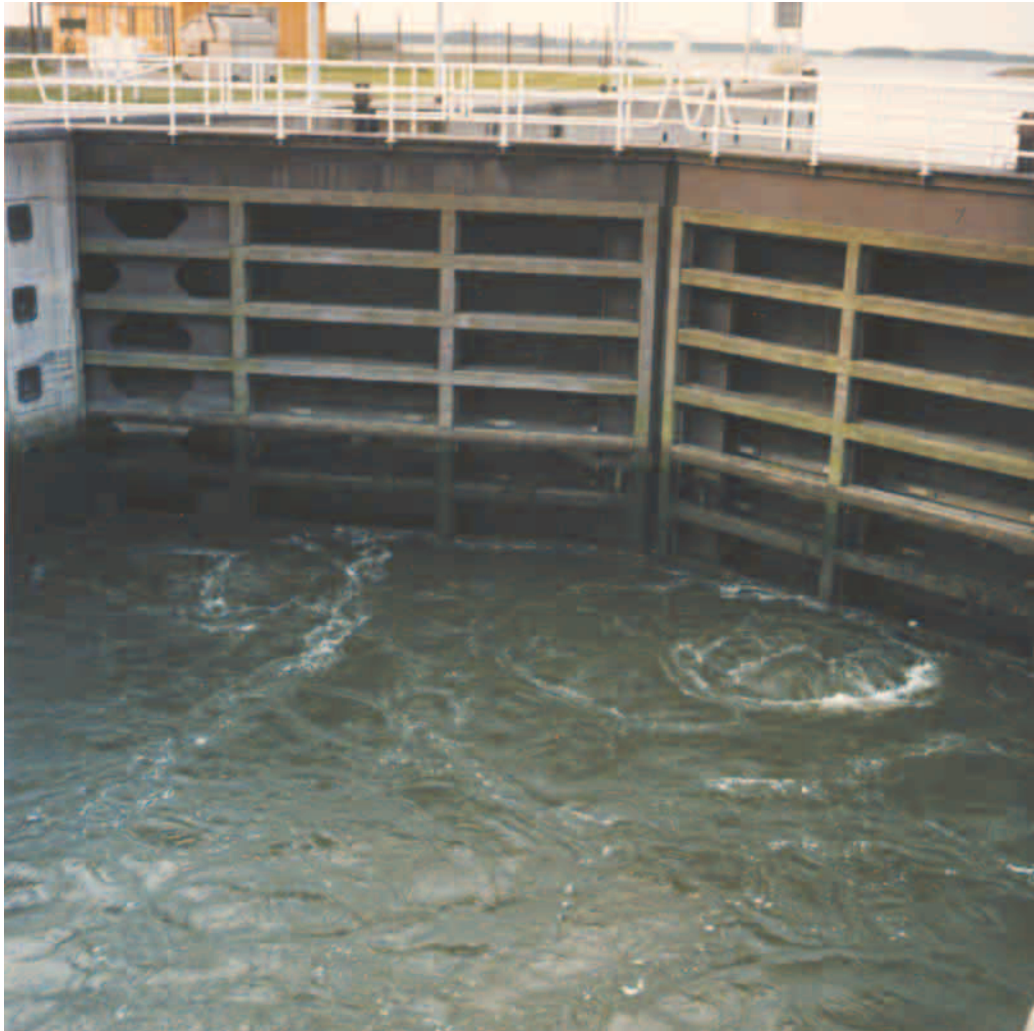
Photo 6.1 Flow pattern during the filling of the yacht lock in the Volkerak
