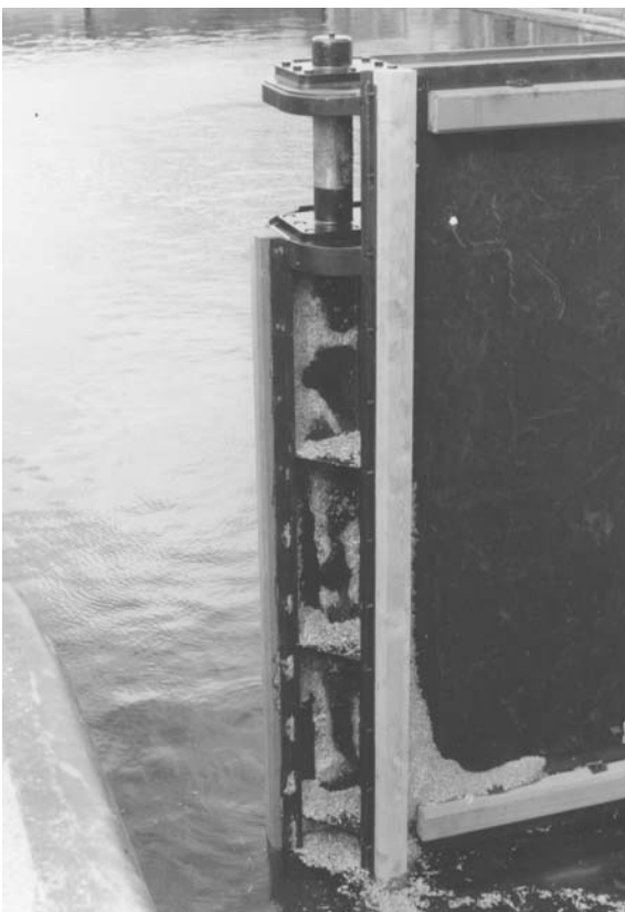
Photo 7.11 Pintle rod of the mitre gate at Middensluis IJmuiden
