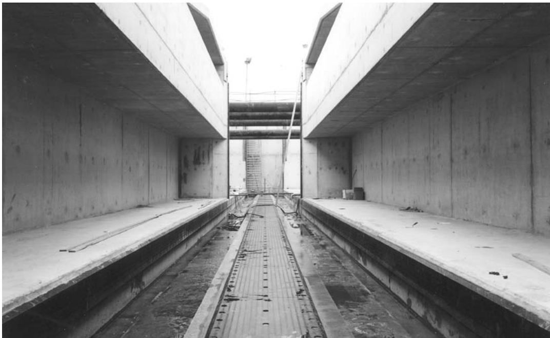
Photo 8.6 Gate chamber of the sliding gate of Nieuwe Oranjesluis in Amsterdam
