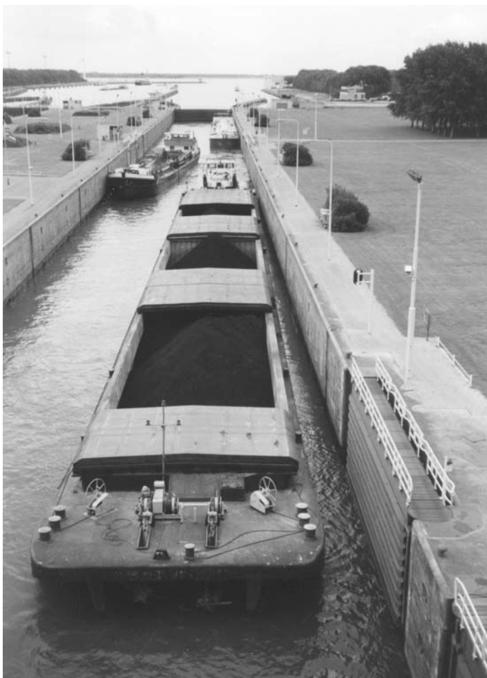
Photo 4.16 Pushed barge CEMT class Va
