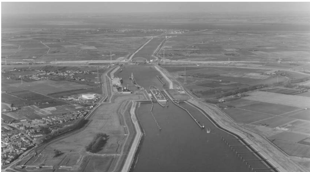
Photo 5.6 Lay out of two push-tow navigation locks in Kanaal door Zuid Beveland
