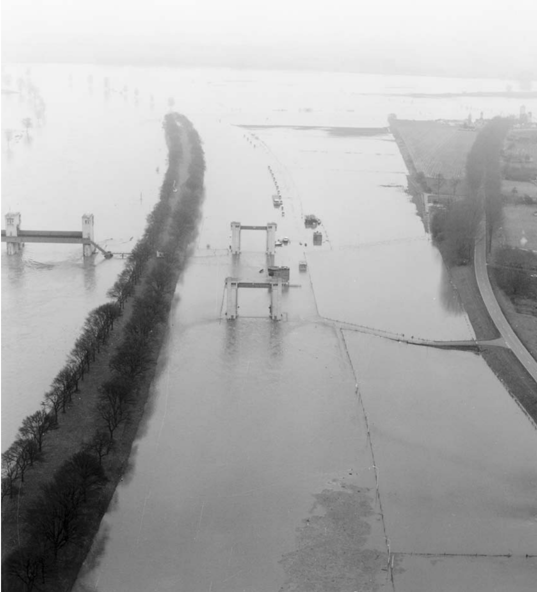
Photo 2.1 Weir and navigation lock complex at Lith during high discharge of the Meuse, 27 December 1993
