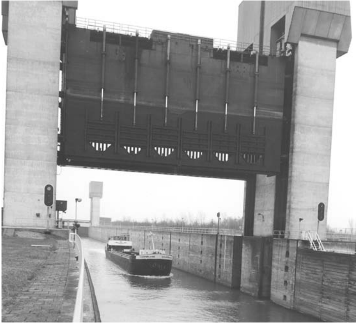
Photo 7.7 Lift gate at Prins Bernardsluis in Tiel
