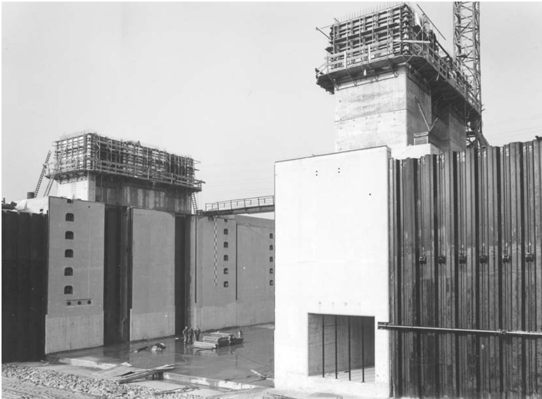
Photo 8.7 Lock head of a lift gate of the Prins Bernard lock in Tiel
