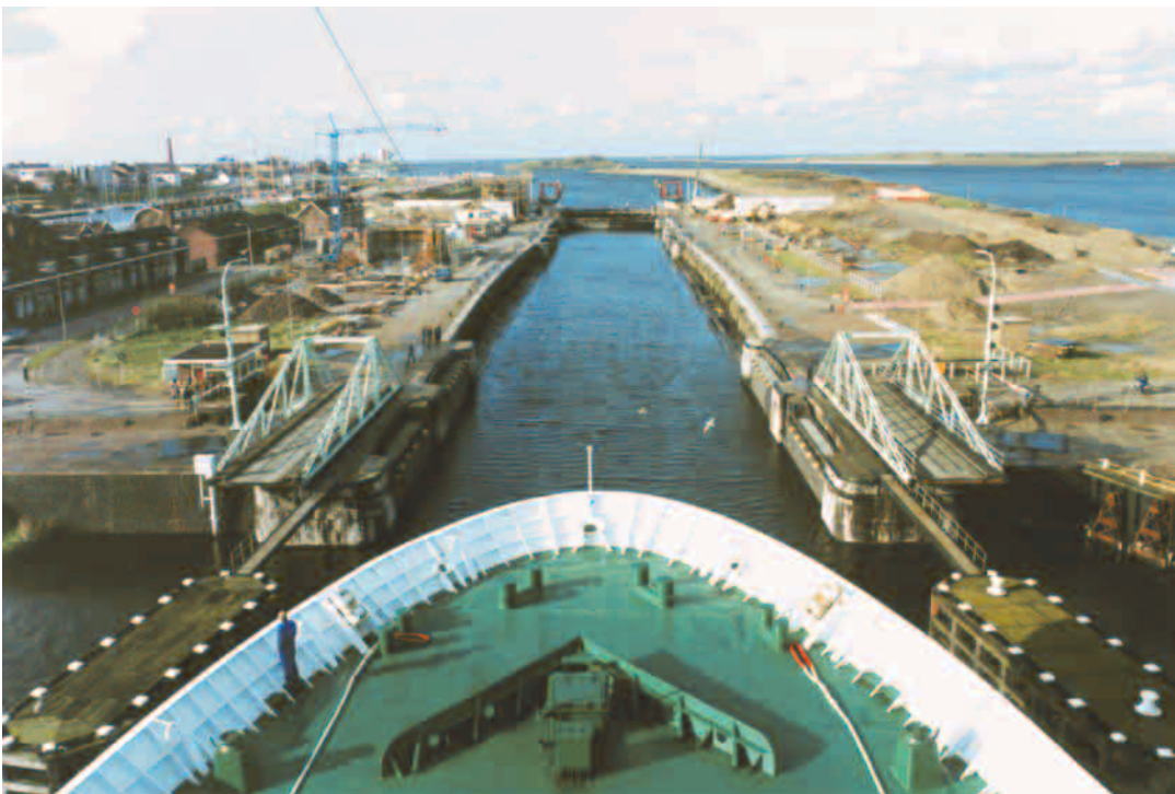
The "Princess of Scandinavia" entering the Middelsluis in IJmuiden (October 1992)
