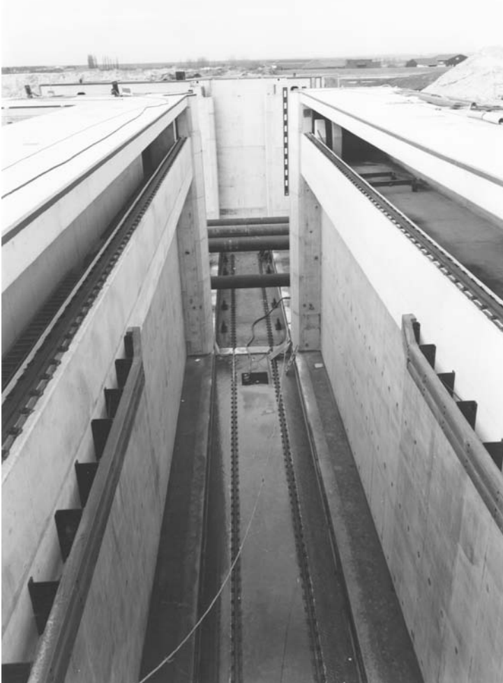
Photo 8.5 Gate chamber of the rolling gate of the push-tow lock in Hansweert
