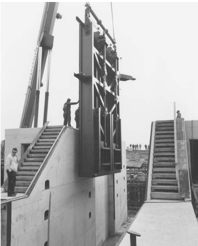
Photo 7.4 Single pivot leaf gate of Lock in Gorinchem (1987)
