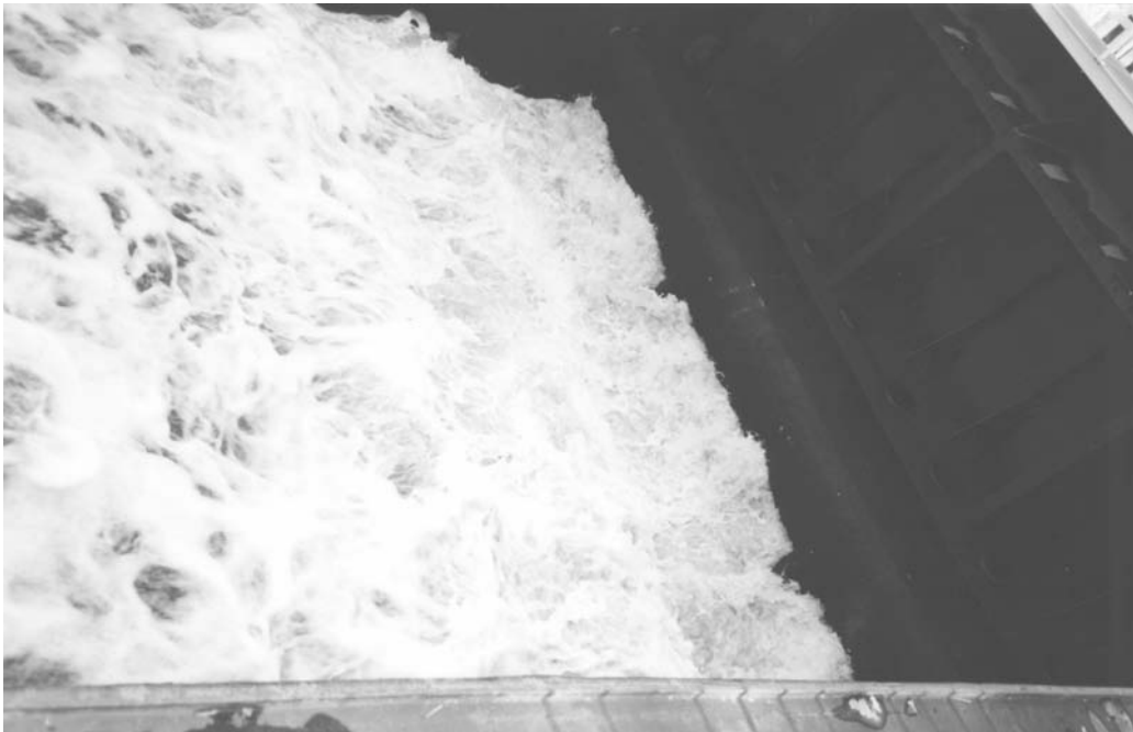
Photo 6.3 Flow pattern during filling by means of lifting the upper gate at the lock in Eefde
