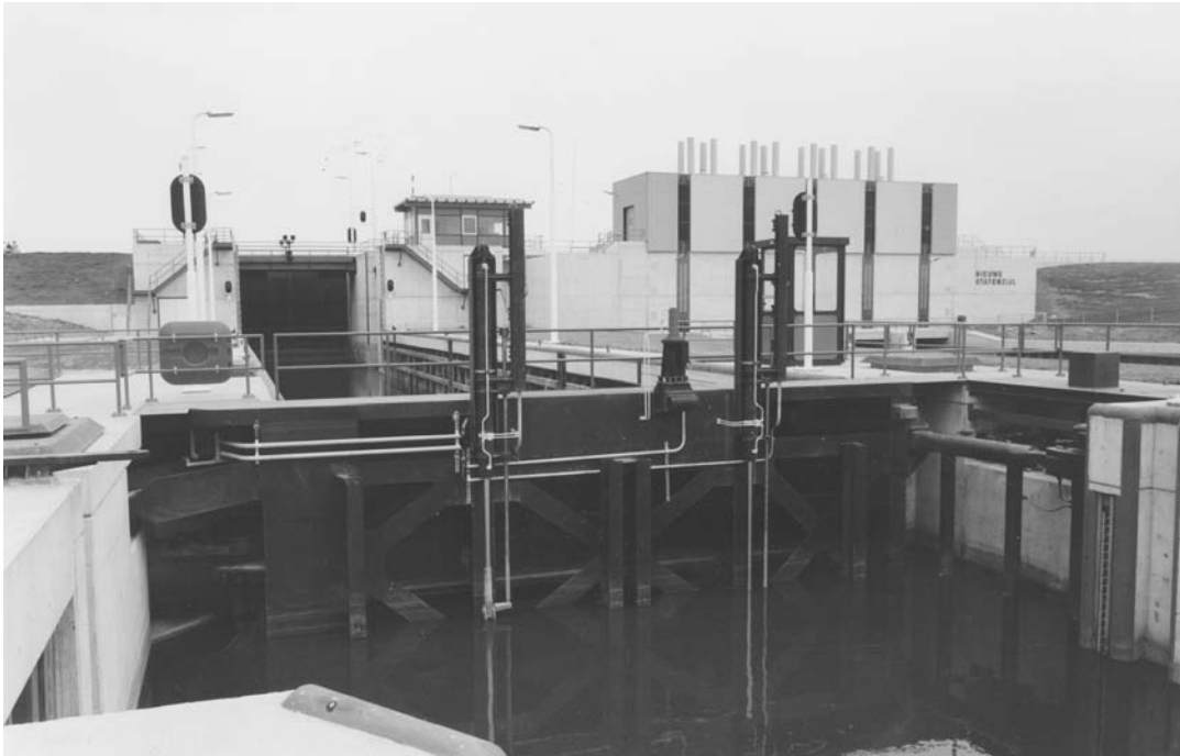
Photo 7.33 Hydraulic cylinder lock paddle operating mechanism of a single pivot gate of the lock at Nieuwe Statenzijl
