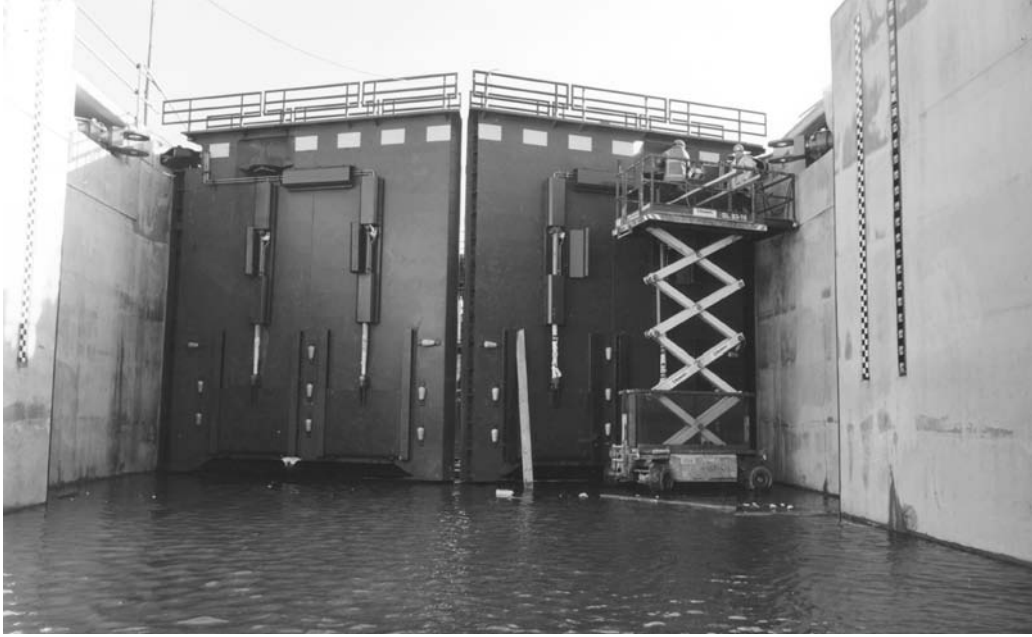
Photo 6.10 Lock paddles for the rectangular openings of the mitre gates of the Kleine Sluis in IJmuiden
