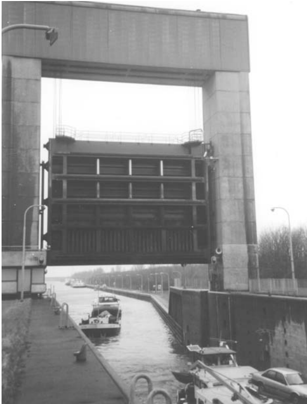
Photo 8.8 Lock head of a lift gate of the new lock in Weurt
