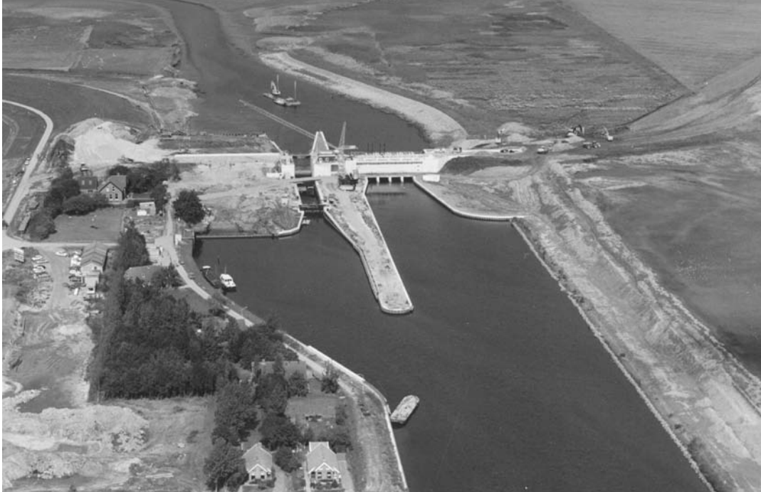
Photo 5.4 Lay out of the lock complex at Nieuwe Statenzijl with navigation lock (left) and drainage lock (right)
