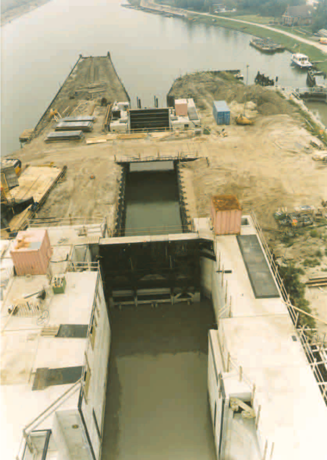
Photo 8.1 Outer head (foreground) and inner head (background) of the navigation lock in Nieuwe Statenzijl
