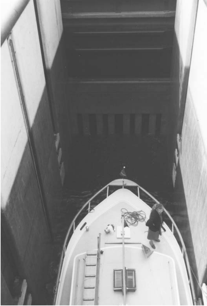
Photo 6.17 Stilling chamber of navigation lock in Almere
