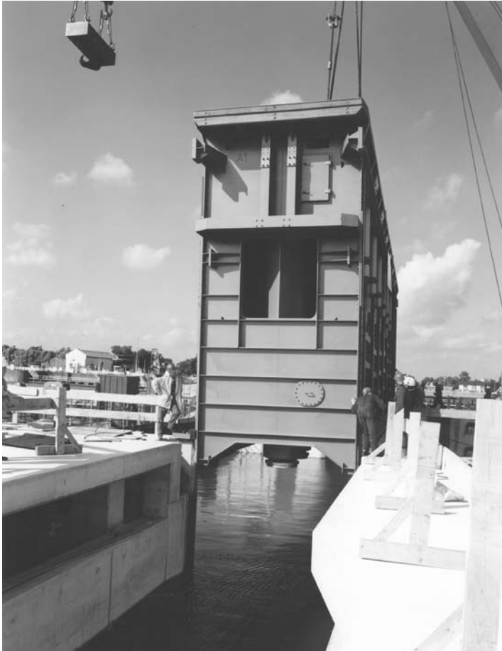
Photo 7.6 Sliding gate at Nieuwe Oranjesluis in Amsterdam during installation (1994)
