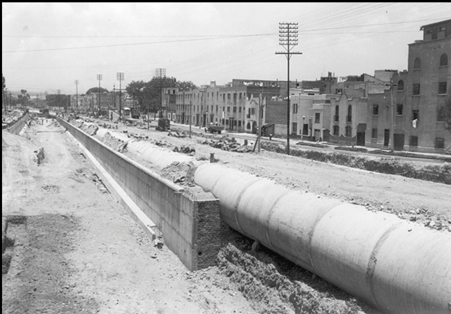
Pipelining of the La Piedad River (Photo: El Universal, n.d.)
