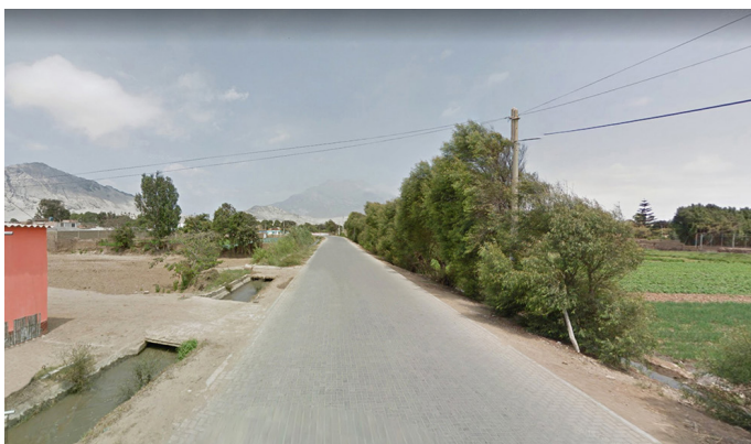
Figure 8.27. The “rural experience”.- before. Source: Google street view image.
