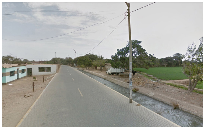
Figure 8.18. The “Countryside belt” -before. Source: Google street view image.
