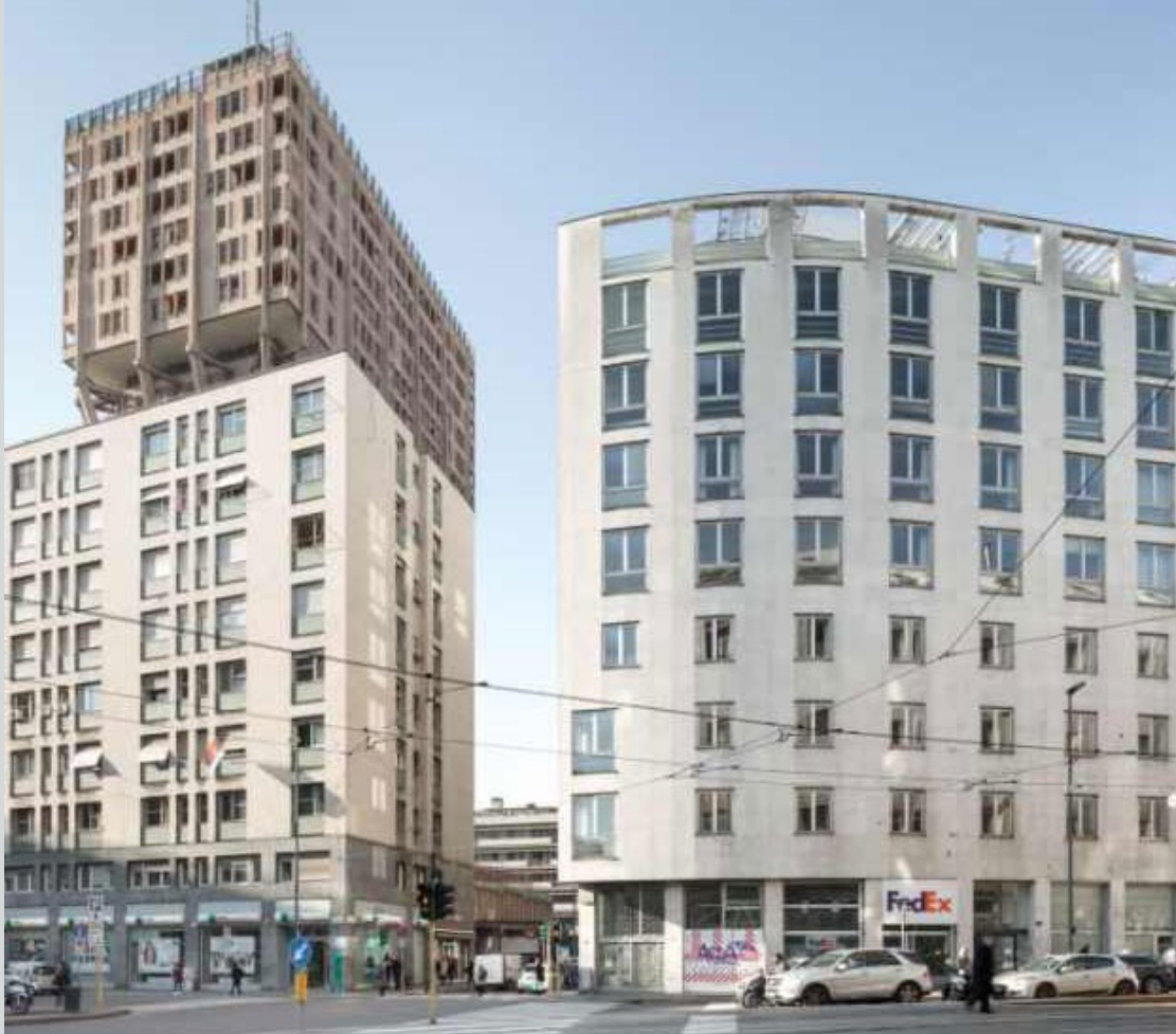
existing structures extended in new architecture by Asagno Vender (Poli, 2014)
