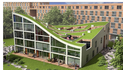
Fig. 1 Residential building “Het Funen” Amsterdam (architect: NLArchitects) with curved cast in site roof
